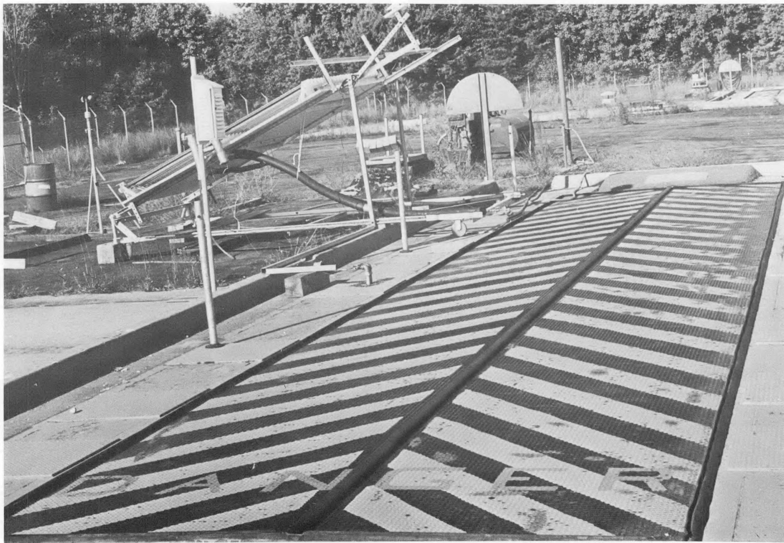
Figure 7 Elevator Door Covering an Underground Storage Bunker at the NIKI Site, NBS, Gaithersburg, Maryland.
