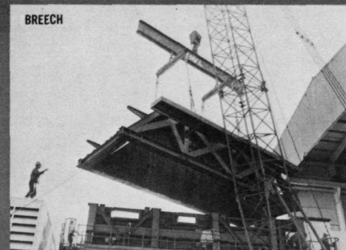
STACK OUTLET DAMPERS
