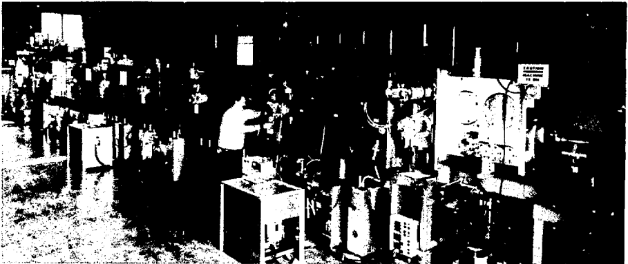
Fig 1 The MBE-4 multiple-beam ion accelerator (CBB 912-117*)
