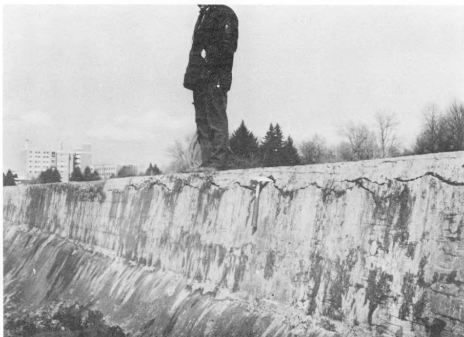
Overflow weir - Note longitudinal cracking on downstream unrestrained surface.
