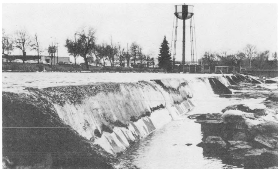
Erosion along weir.
