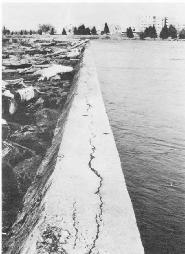
Overflow weir - Note Longitudinal cracking along crest.
