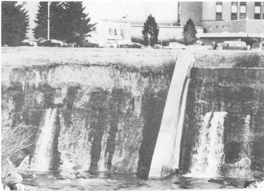
Seepage through weir - Note boil on downstream side (lower left of photo).
