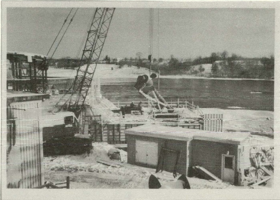
9. Unit #7 Runner and Shaft Assembly January 25, 1982
