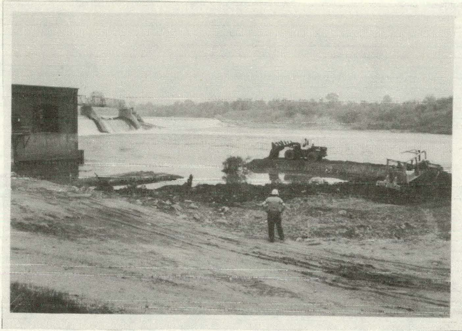
1. Earth Cofferdam Construction June 4, 1981
