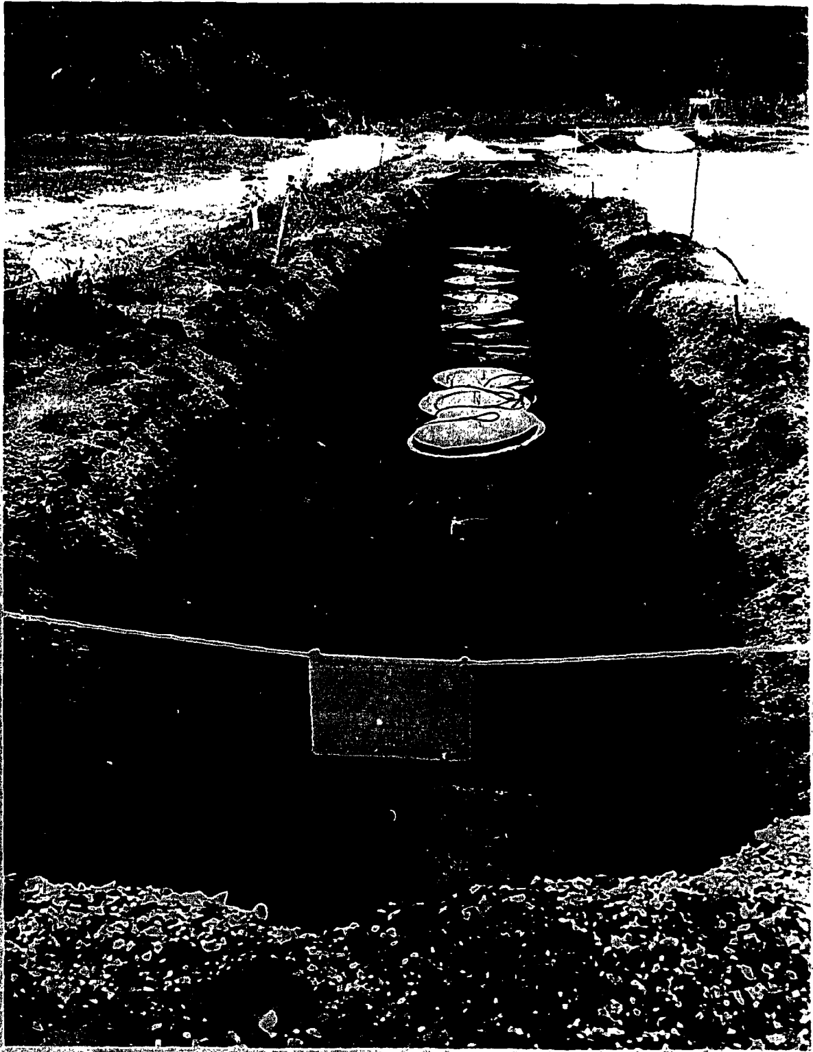
Fig. VI-4. Concrete casks used for TRU wastes with high external gamma exposure rates.
