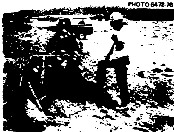
Fig. 9.6. Collapsed entrance facing away from ground zero, at 15 psi. The blast winds had scoured away most of the covering earth, and the earth had "flowed" away from the center of the shelter, pushing the upper part of the entry in a direction perpendicular to the radius from ground zero.
