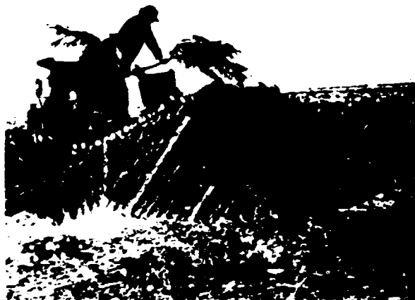
Fig. 9.3. Covering the frame of a Ridge-Pole Shelter with salt cedar limbs.
