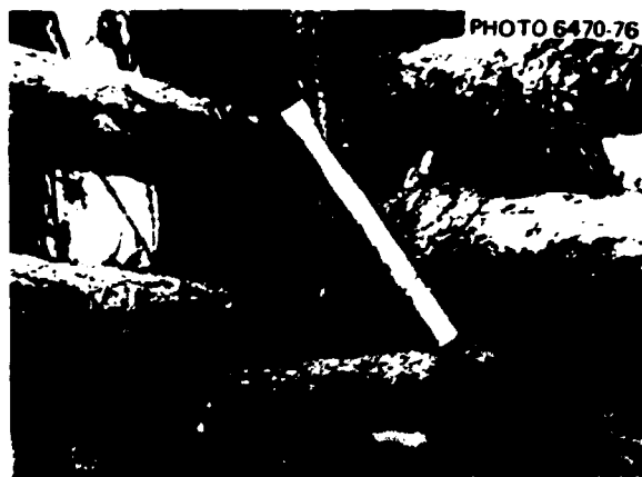
Fig. 11.9. Postshot condition of the lightly constructed triangular vertical entry. The hammer rests on a step pole. Earth arching prevented the yielding bed sheet outside from being torn.
