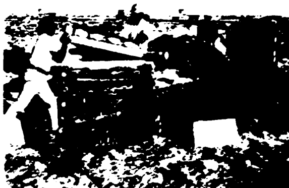
Fig. 11.2. Completed frame of Chinese "Man" Shelter tested at 20 psi. In accord with the Chinese drawing, the poles of the main room averaged only about 3 in. in diameter. The triangular entries and triangular blast doors were of ORNL designs.
