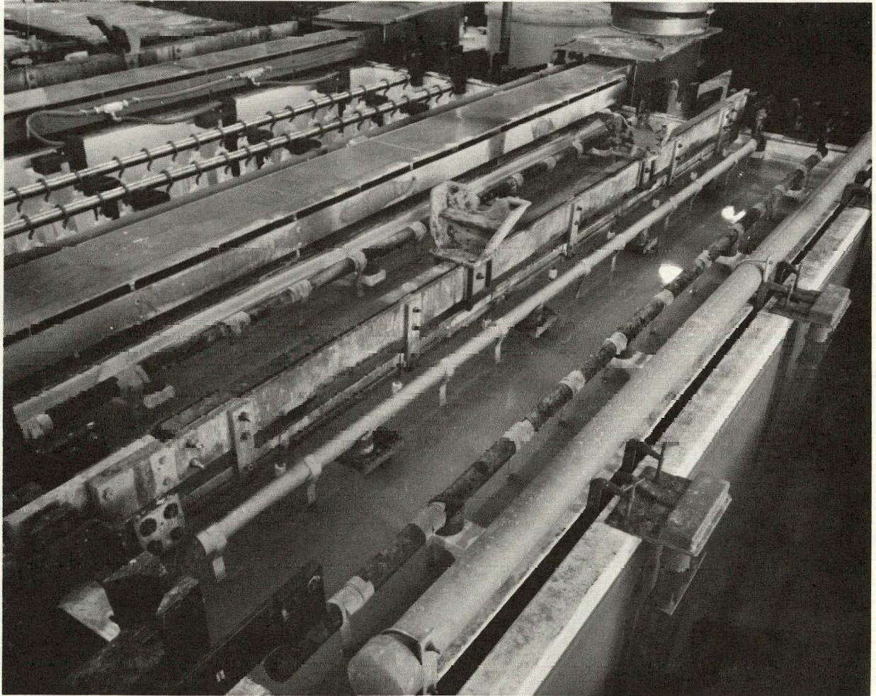
Figure 2.10 MAXI-LINE FORMATION TANK (CENTER)
