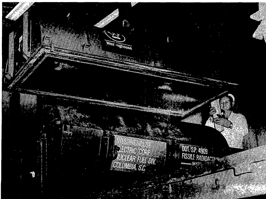
Fig. 1. 2-1/2 ton UF_6 cylinder overpack - horizontal loading type.
