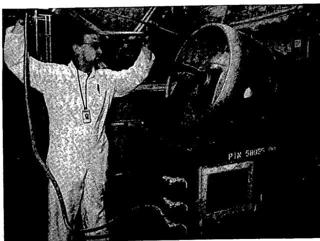
Figure 9 Steam Lance Inserted
