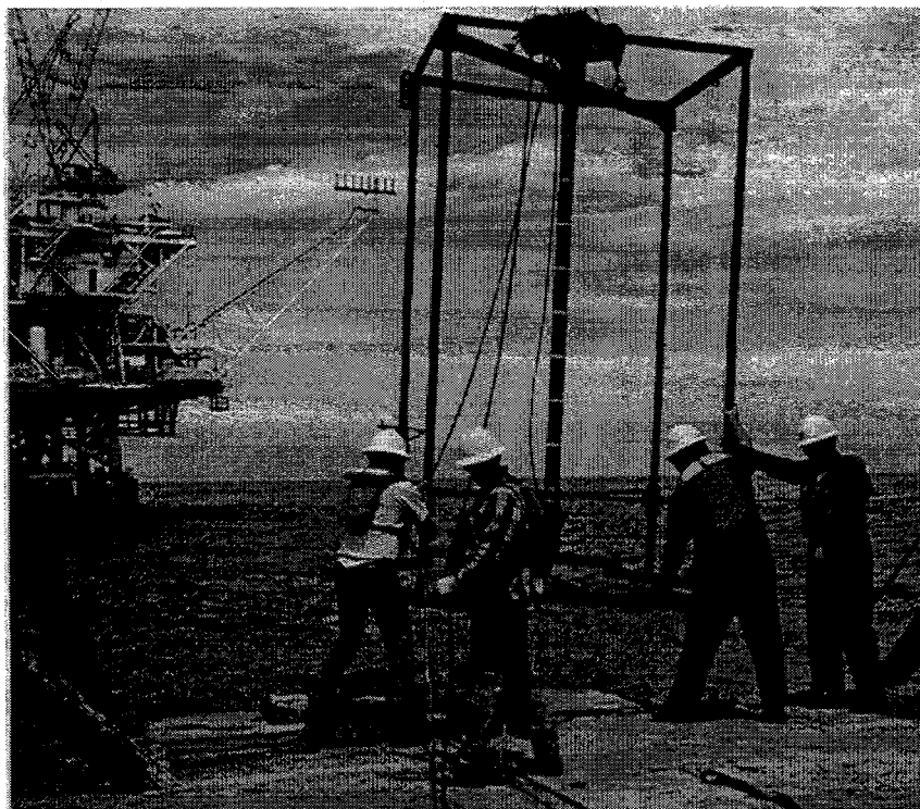
Figure VI: View of Installation Cage as it is lowered over the boat
