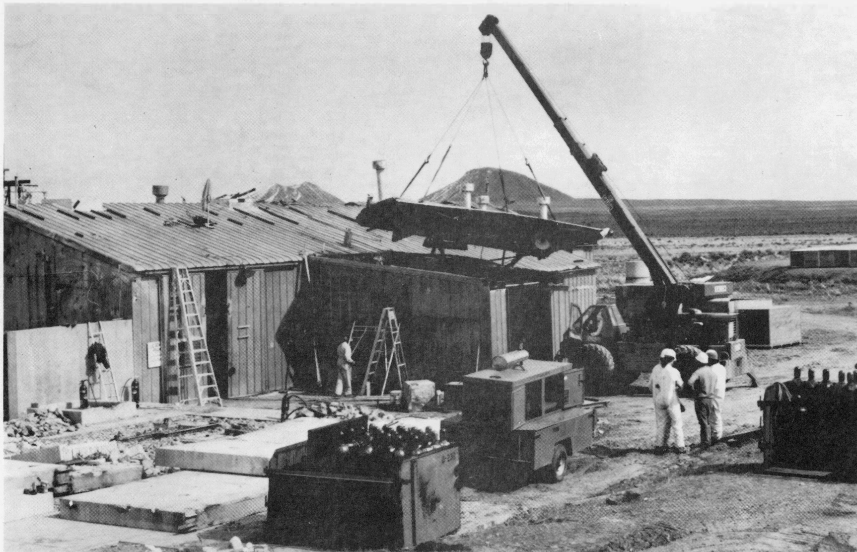
Figure 42. Removing part of the process and control building.
