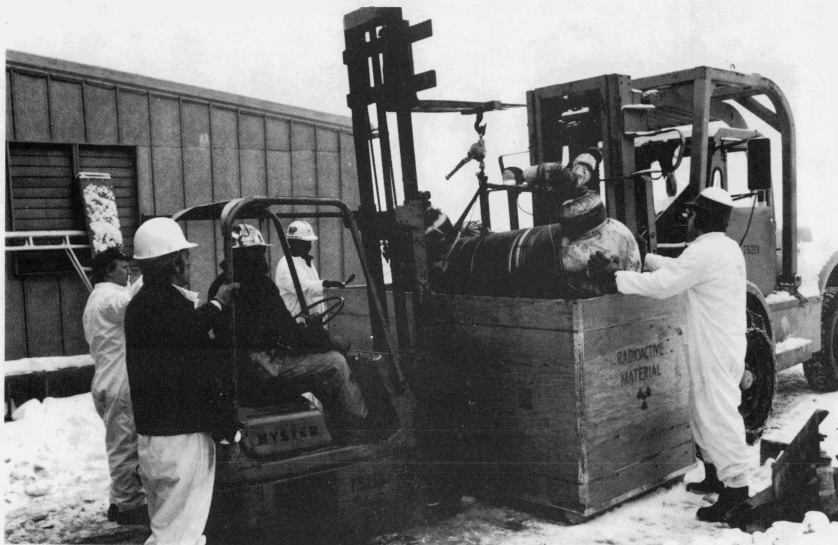
Figure 69. Contaminated tank placed in plywood box.
