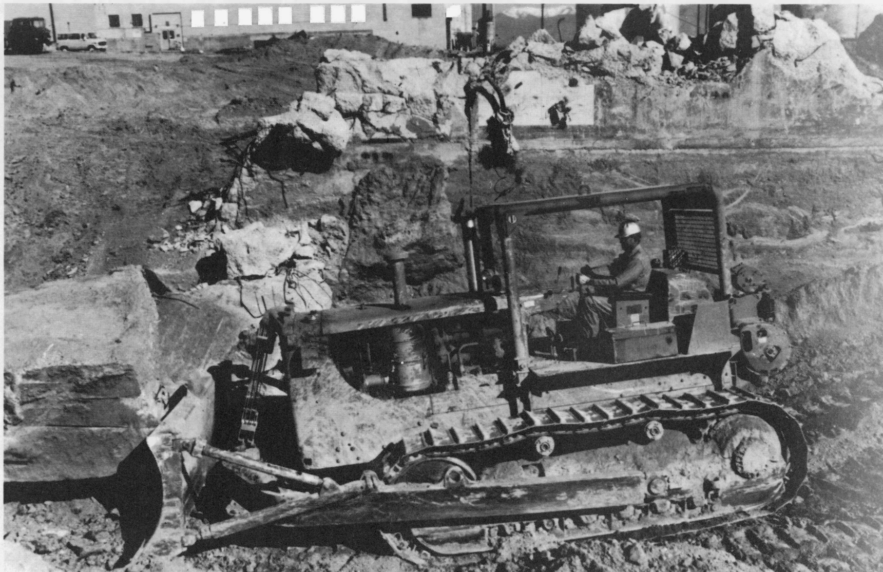
Figure 57. Digging a pit at the foot of the shield wall.
