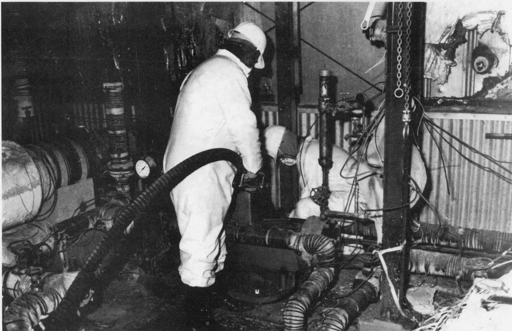
Figure 27. Removing asbestos insulation from piping prior to cutting pipe.
