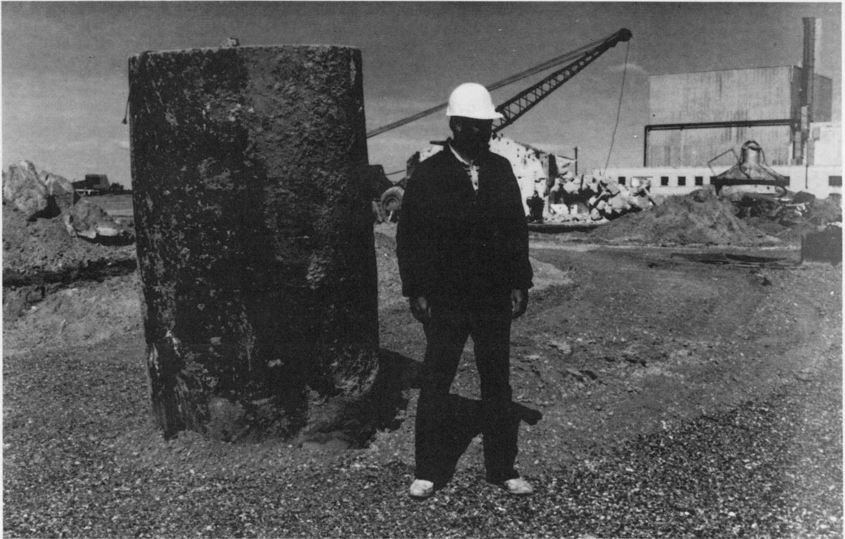
Figure 47. Contaminated waste water tank excavated from under cordox system concrete slab.
