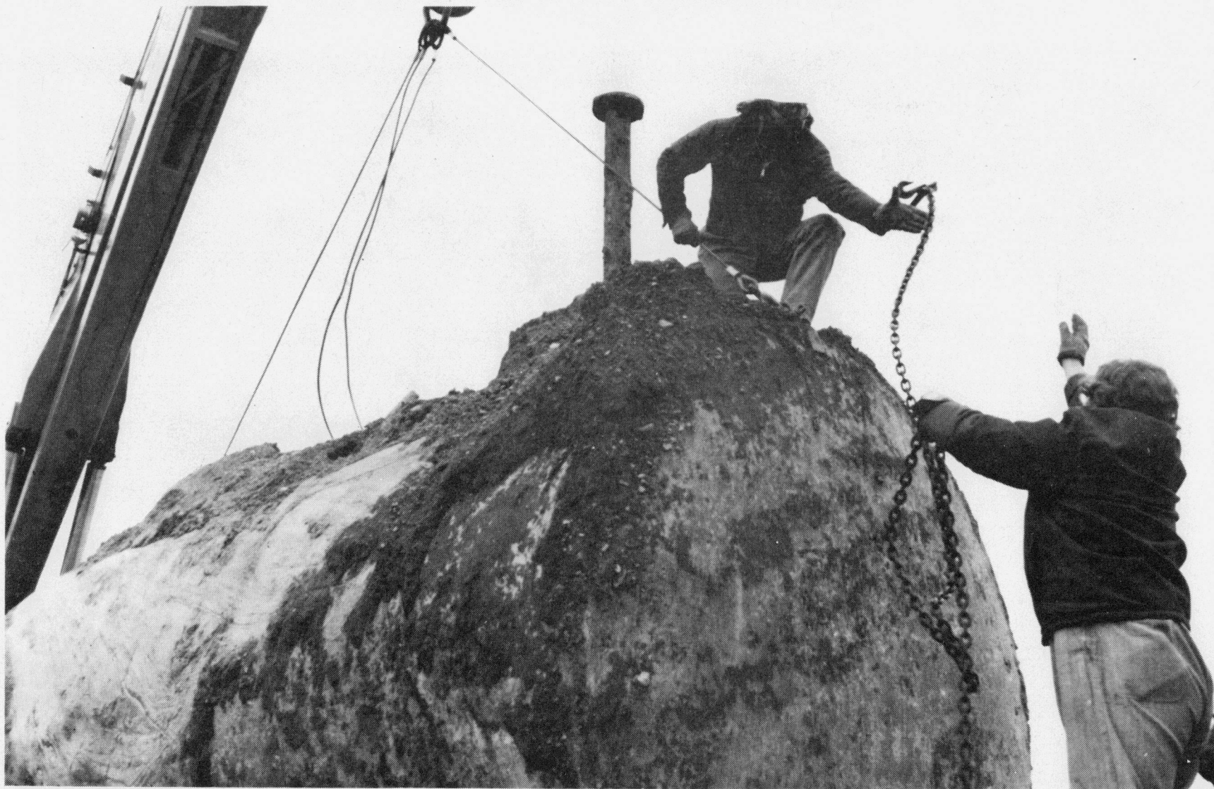
Figure 46. Rigging to xylene storage tank.
