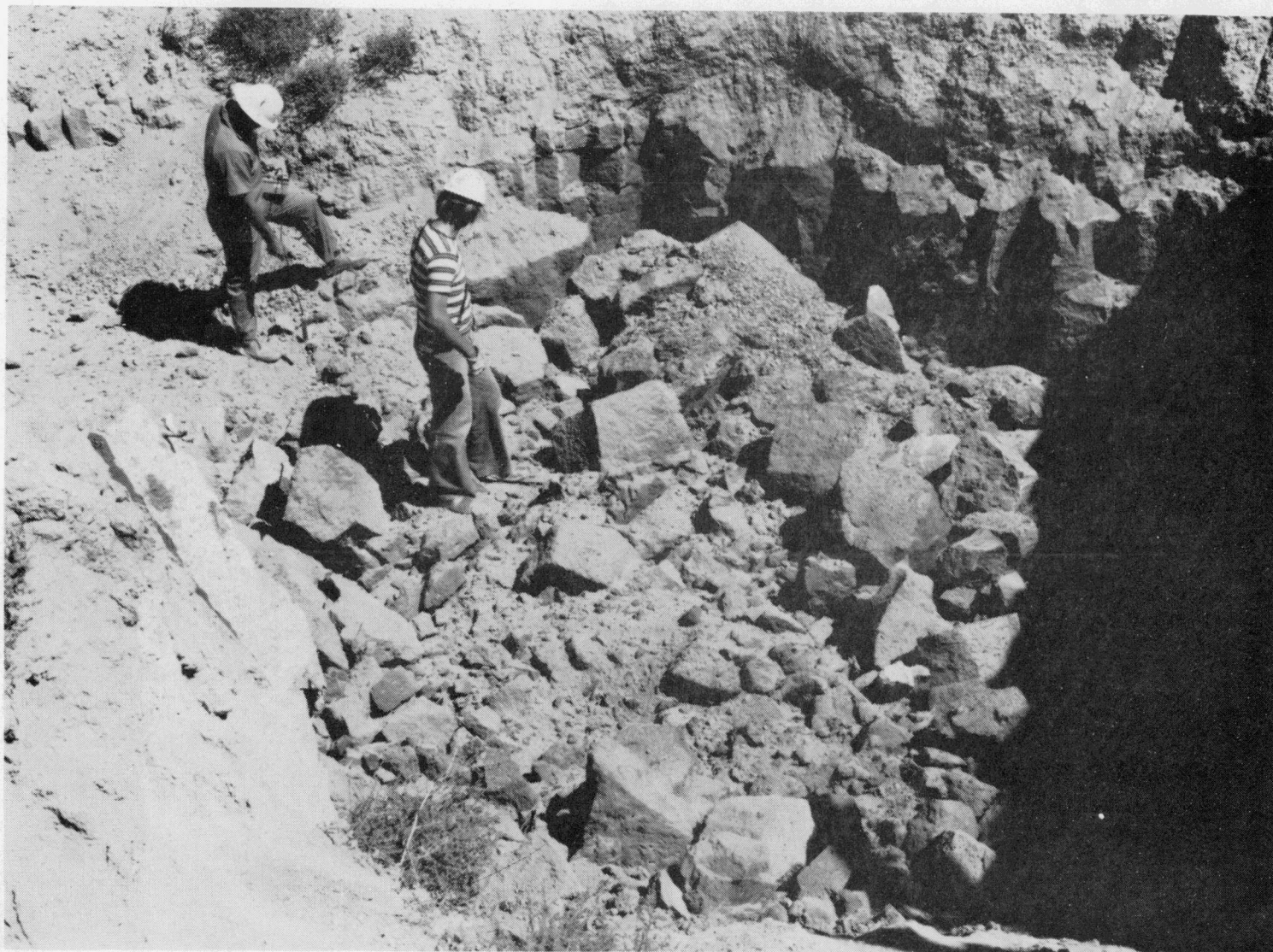
Figure 68. Basalt rubble after blasting.
