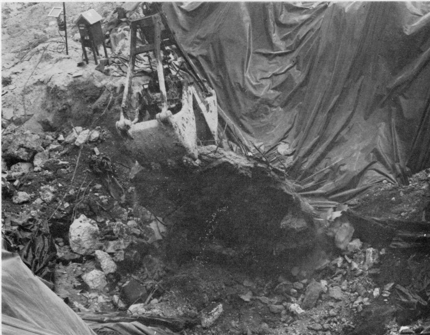
Figure 66. Remnant of reactor pad loose from basalt.
