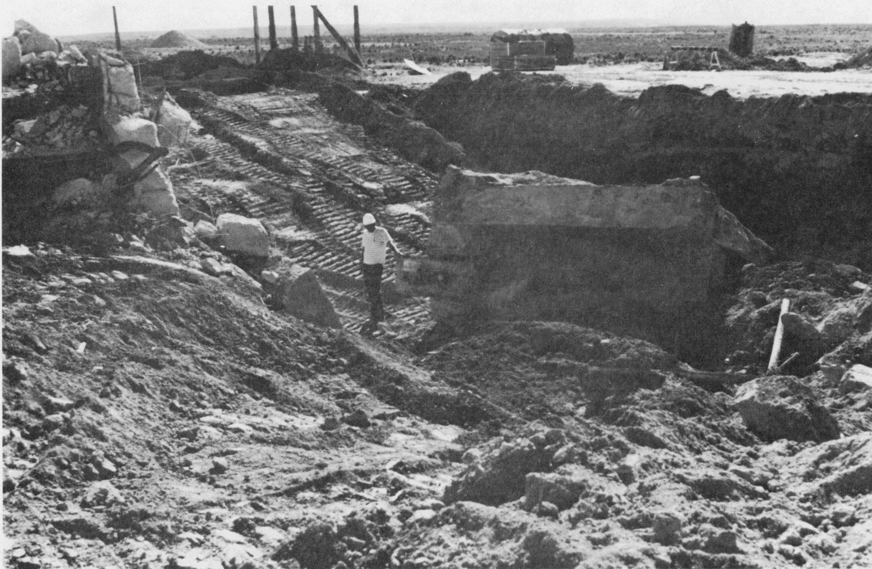
Figure 54. Burying parts of the uncontaminated shield wall.
