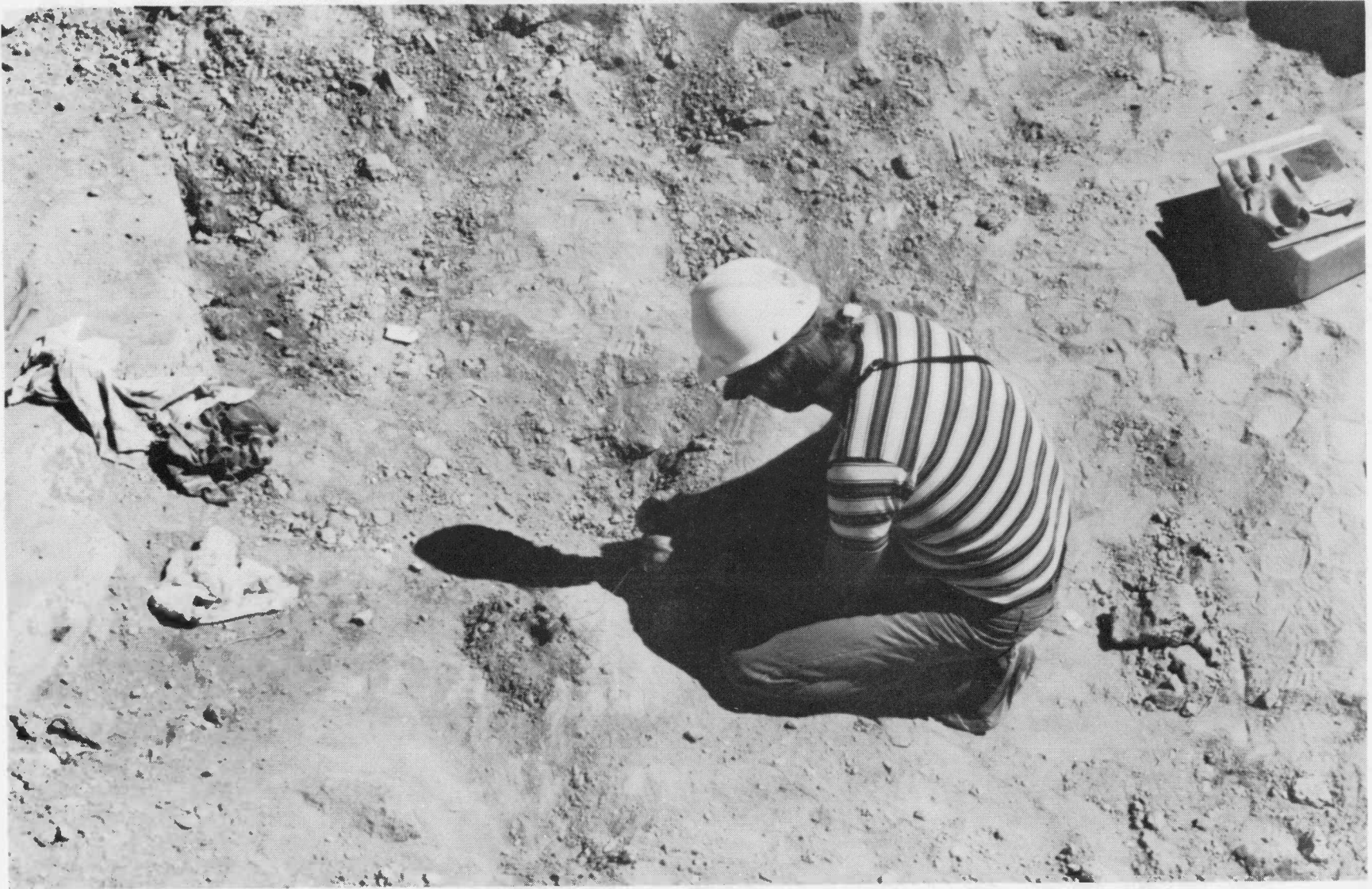
Figure 67. Setting charges in excavation basalt.
