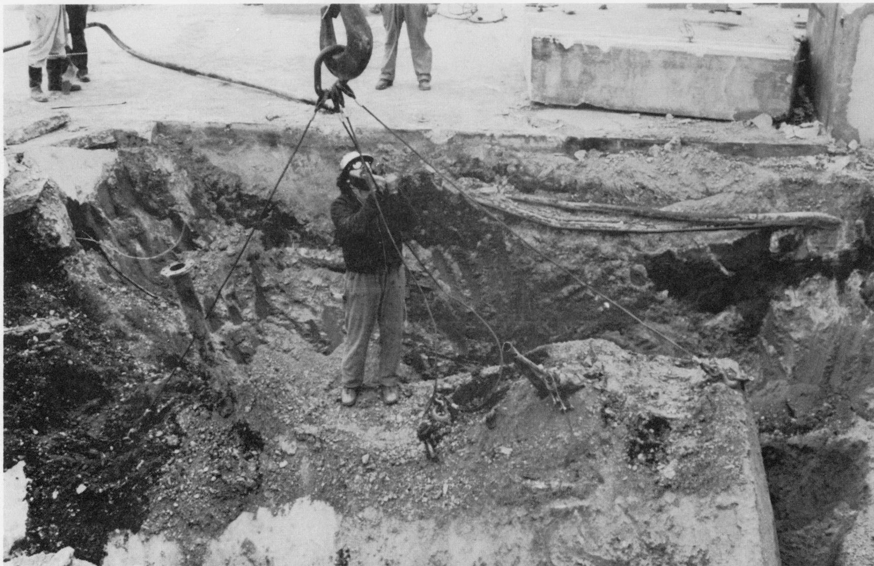
Figure 48. Rigging to the liquid waste tank.
