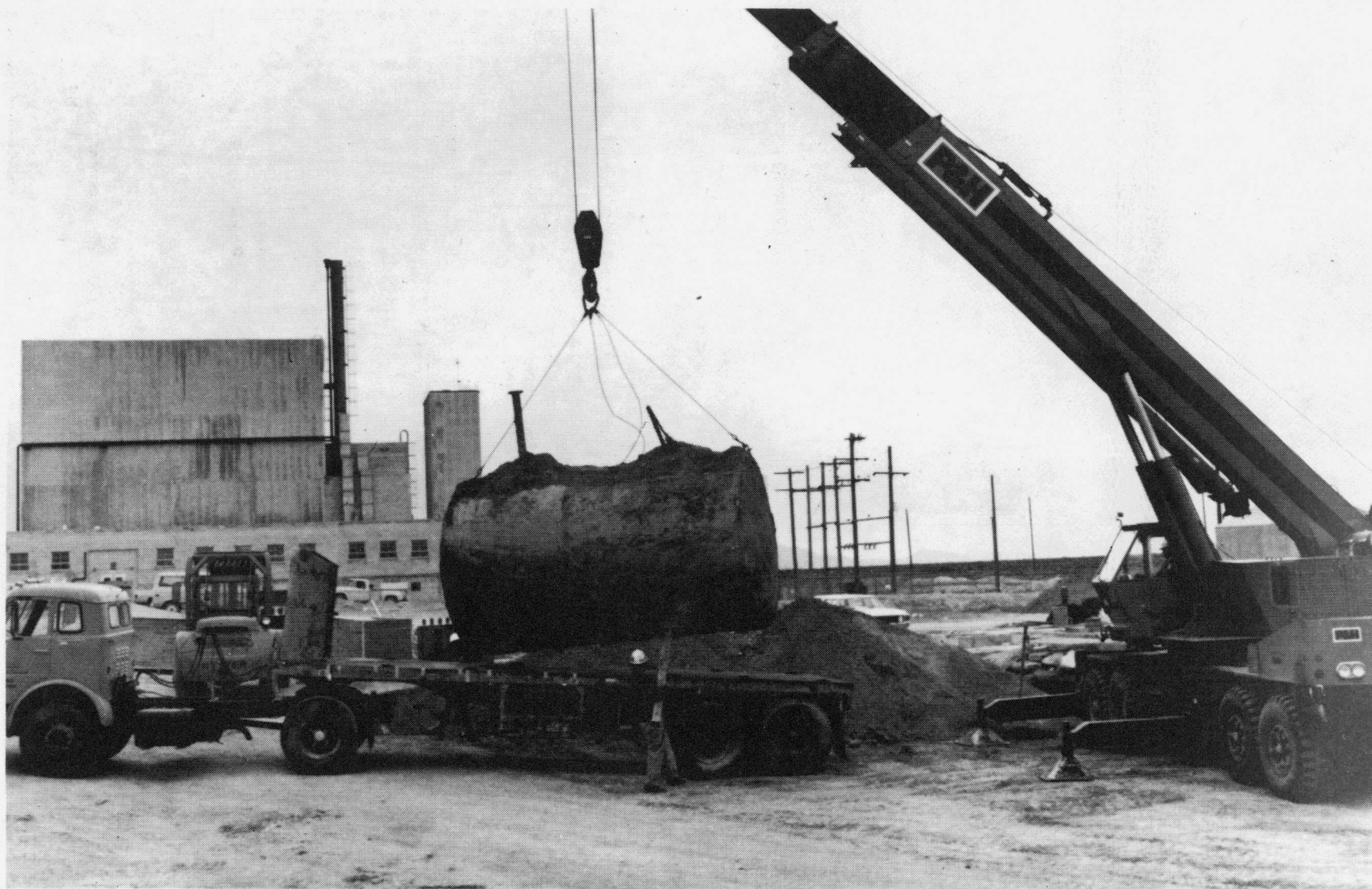
Figure 51. Setting liquid waste tank on lowboy.
