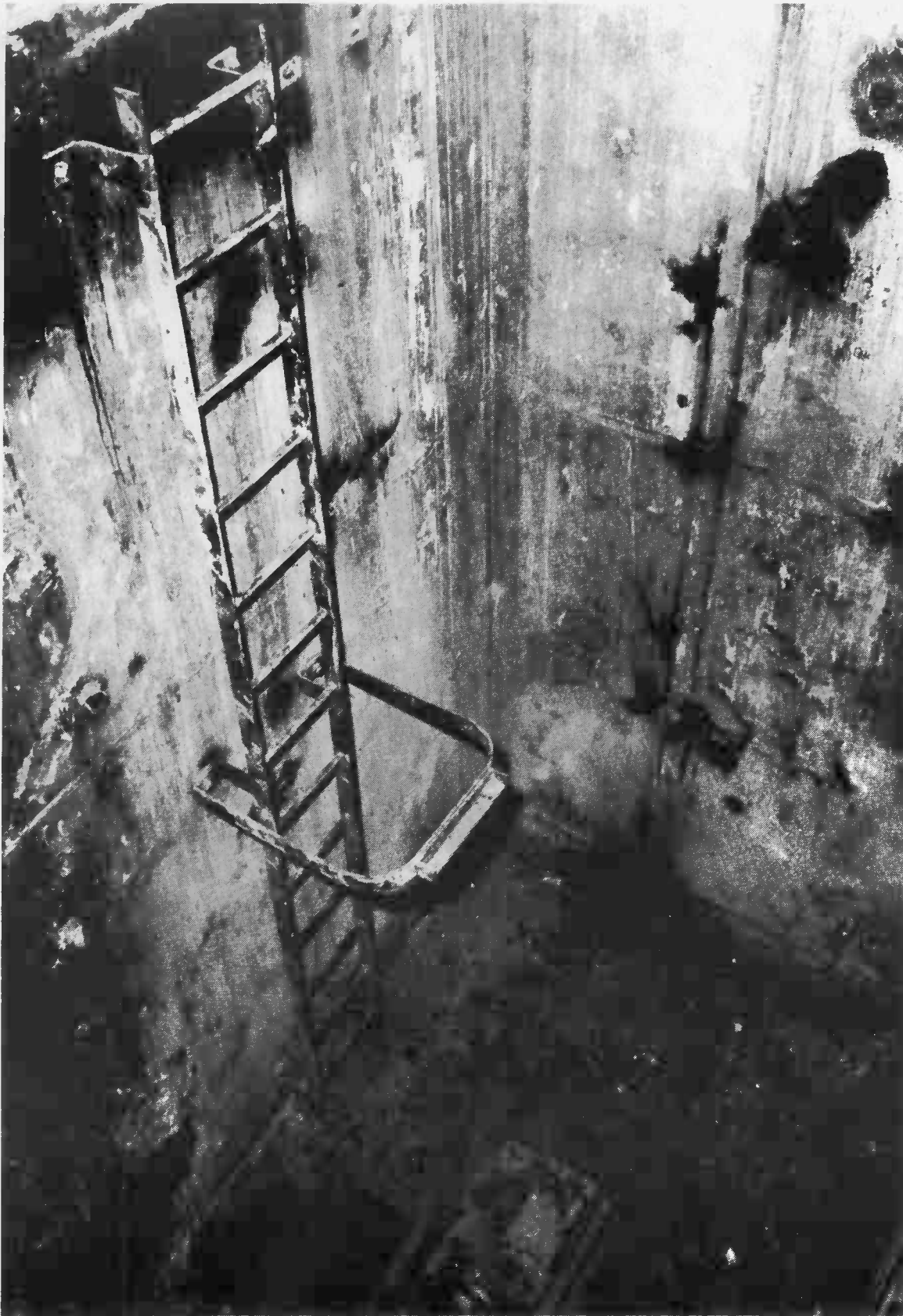
Figure 31. Process and control building pit after removal of purification system piping.
