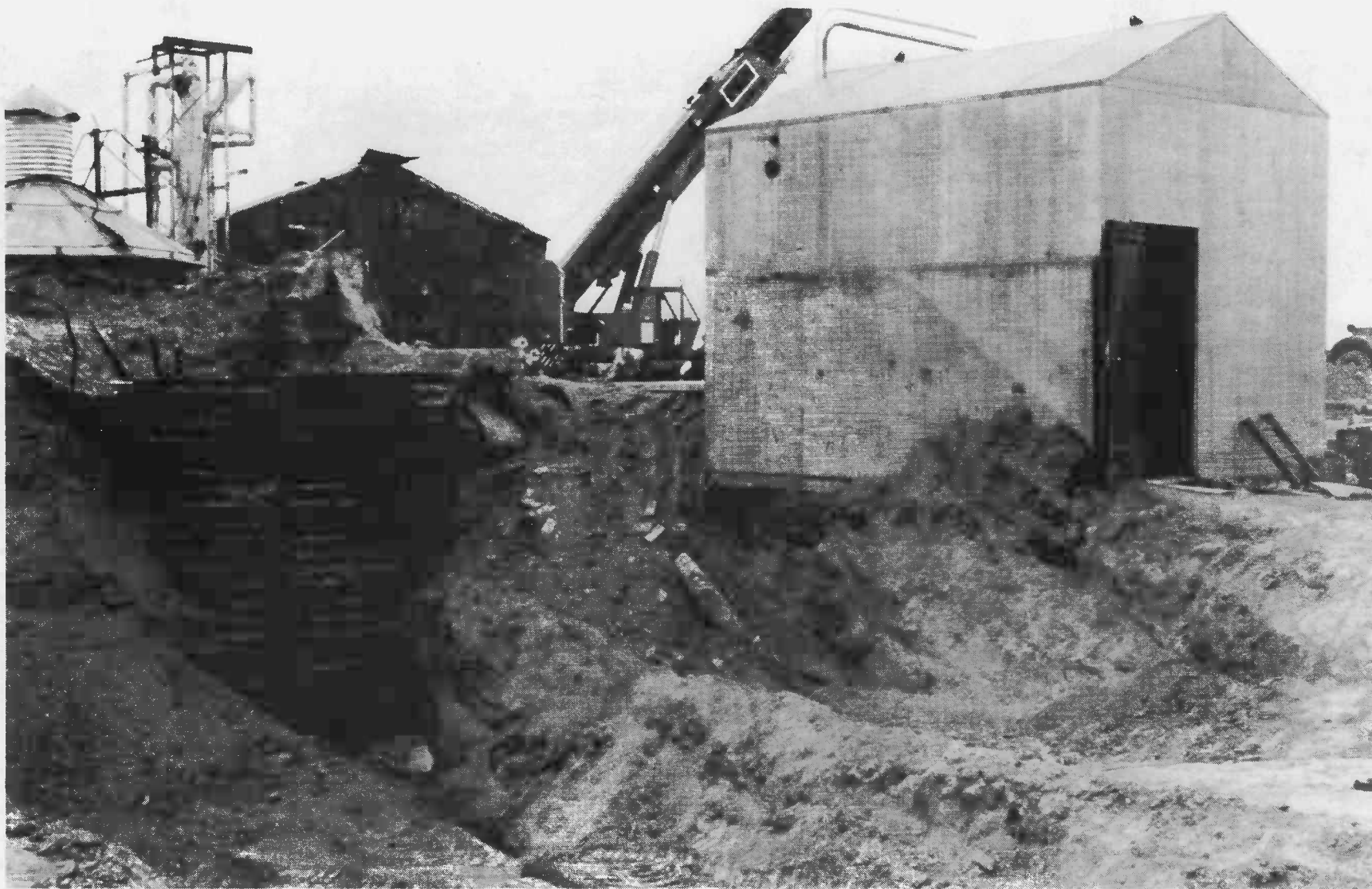
Figure 59. Exposed pipe gallery silo concrete cover slab removed.
