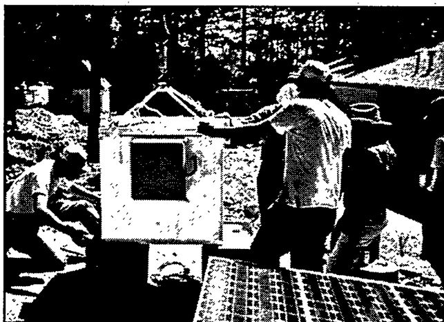
The PSREC residential system enclosure is lifted onto its foundation
