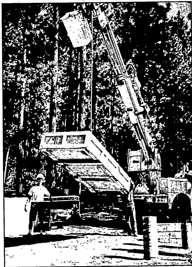
Crated array is unloaded with PSREC's boom truck.
