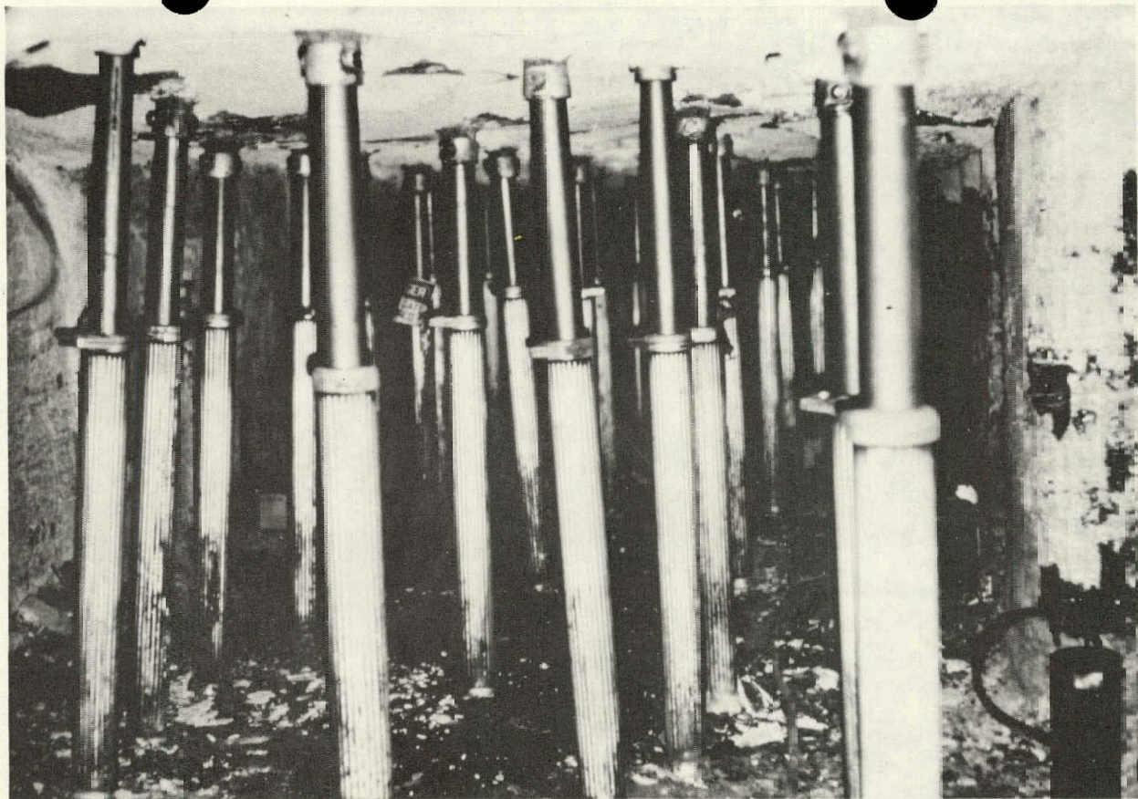
FIGURE 11. - Props in Supply Gate
