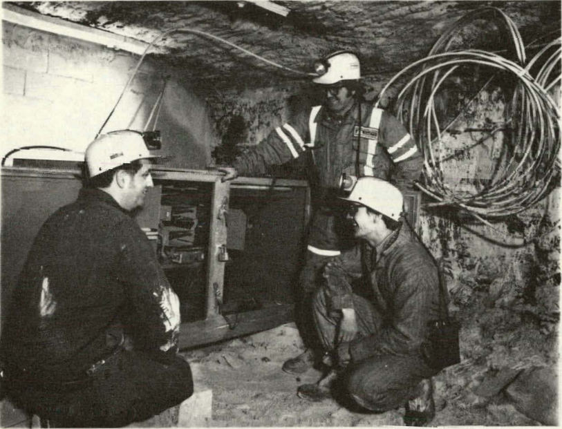
FIGURE 5: TYPICAL INSTALLATION OF TELEMETRY STATION
