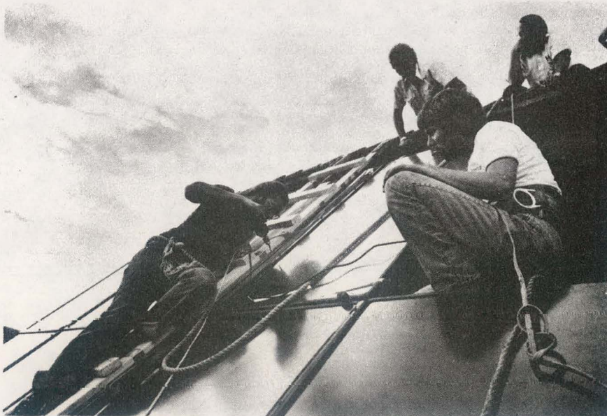
Figure 2-14. Cap Strips Placed between Adjacent Collector Modules
