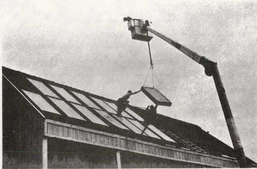
Figure 2-11. Installation of the West Collector Array in Solar House II
