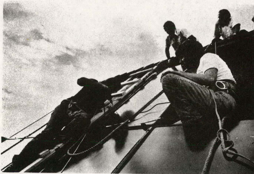
Figure 2-20. Attaching Cap Strips with Better Procedure
