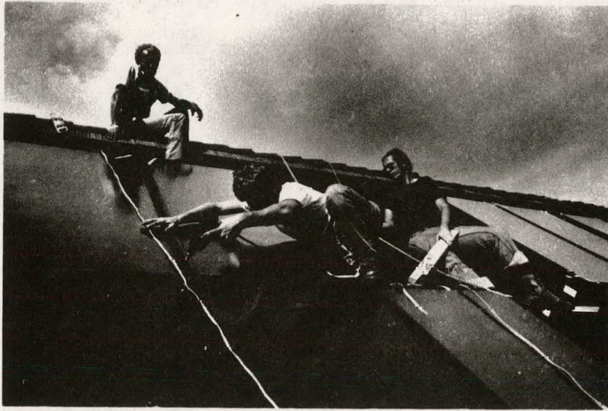
Figure 2-19. Attaching the Cap Strips between Collector Modules
