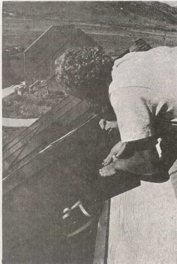
Figure 2-18. Flashing was Installed Around the Entire Array
