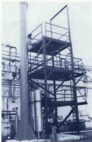
Figure 2. Tall Reformer Tube Test Facility
