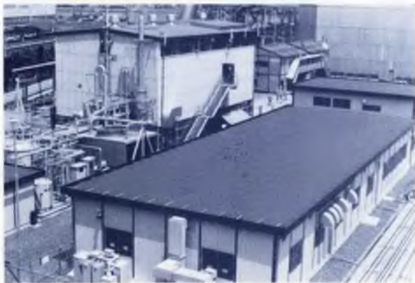
Figure 1 Outline of the pilot plant
