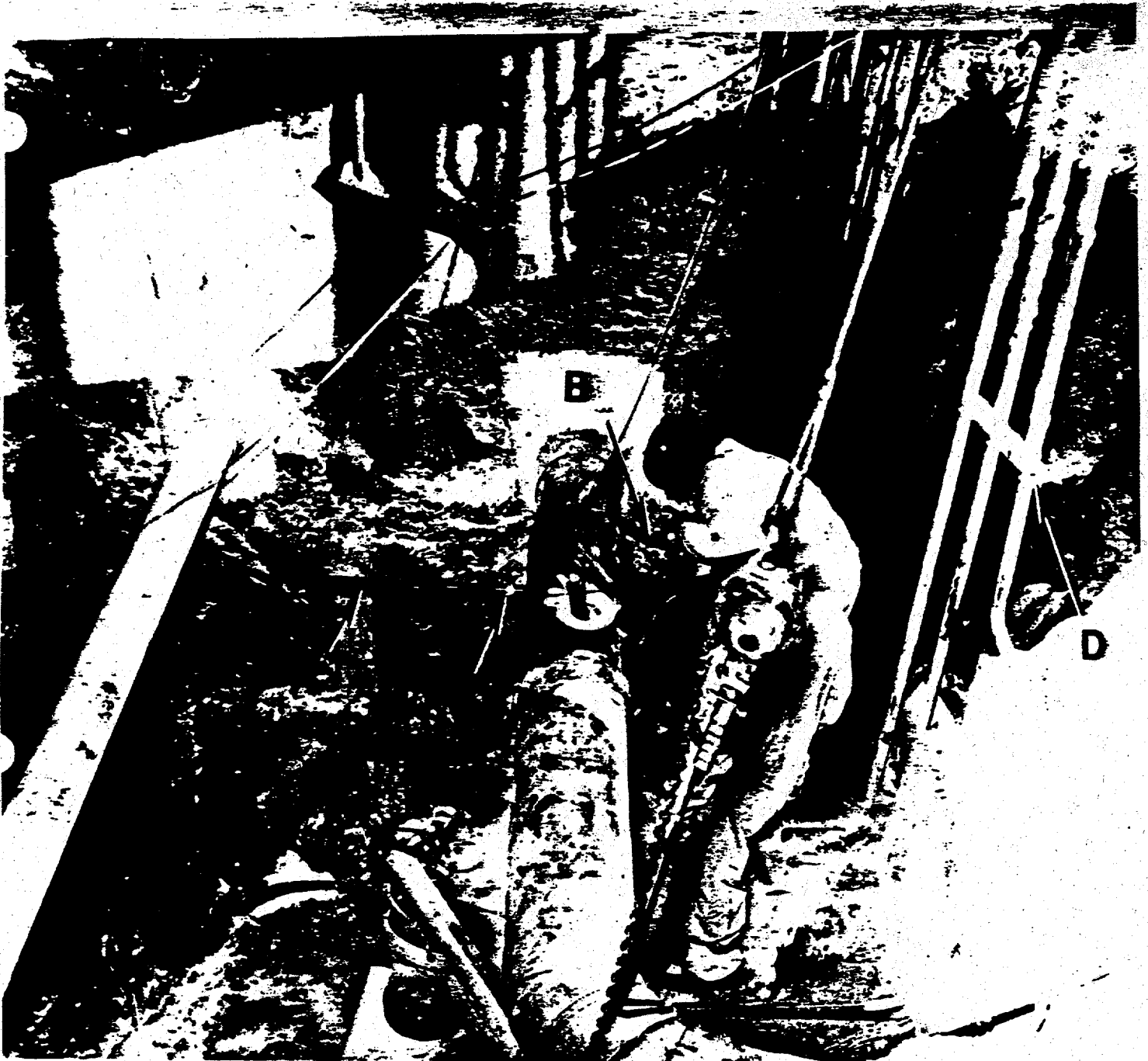
Figure 3. Large excavation at leak site. Hole C in the leak detection system drain pipe occurred at the interface between two backfill materials having very different electrical properties.
