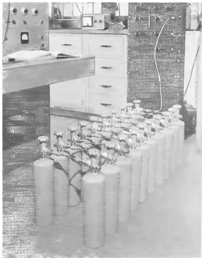
Figure 4. Filling twenty small cylinders from master mixture.
