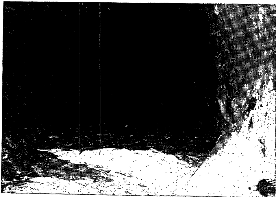
Figure 20. Pillar Decay by Slabbing in Rooms. Intersection G8 of Upper Level.
