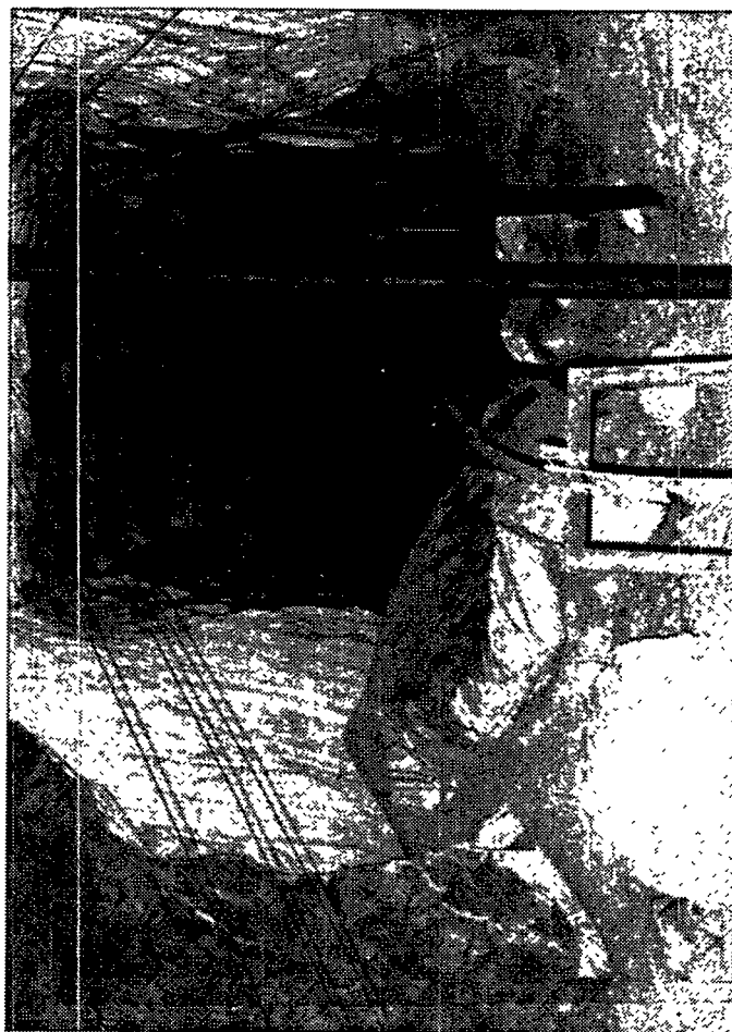
Figure 28. Piles of Ravelled Salt from Exfoliated Pillars. Intersection E7 of Upper Level.
