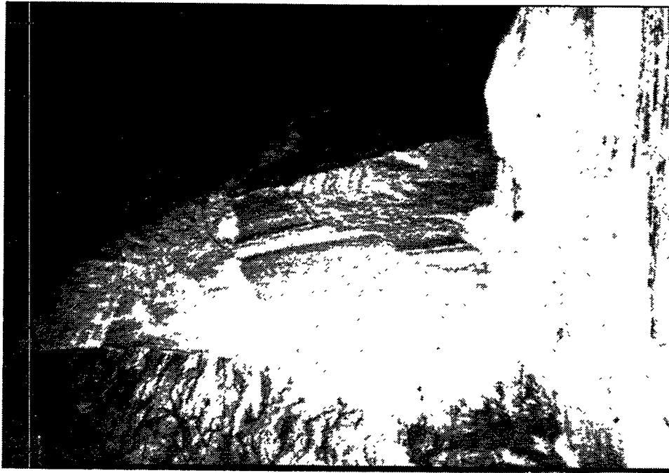
Figure 26. Piles of Ravelled Salt from Exfoliated Pillars. Room A Between Crosscuts 5 and 6 of Upper Level.
