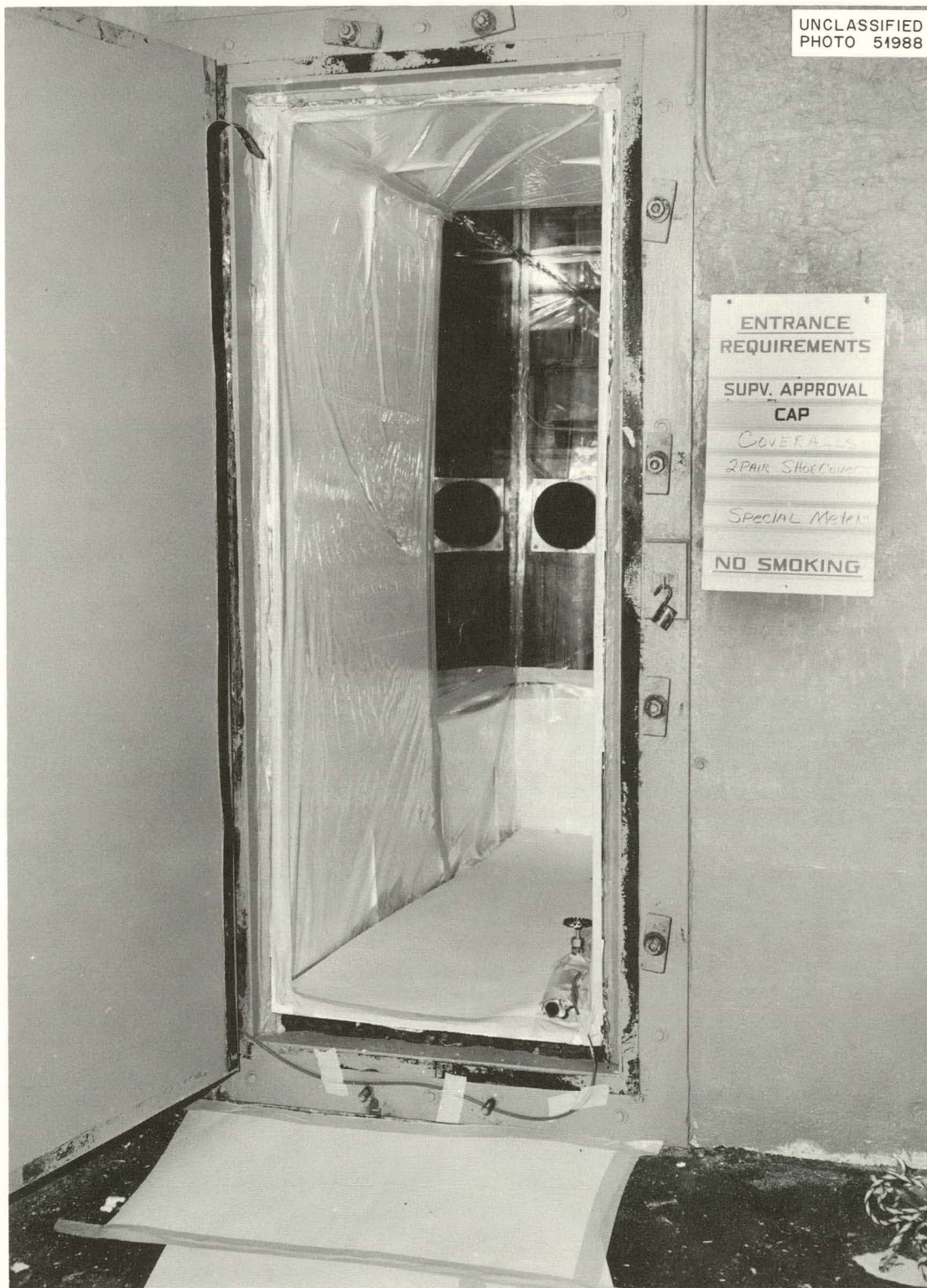
Fig. 6.1. View of Temporary Cubicle from Plenum Chamber.
