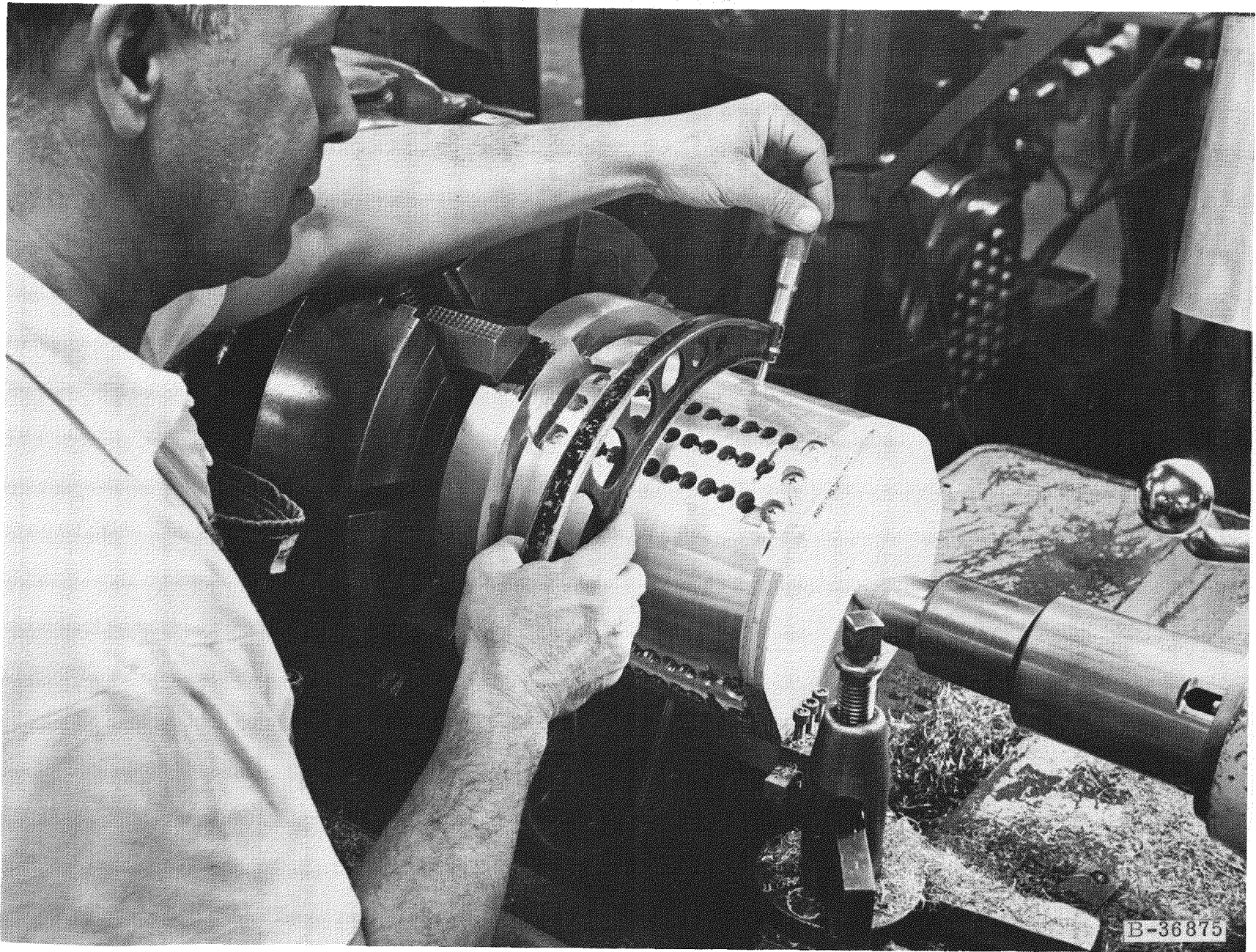
Fig. A-2. SNAP 7A and 7C Heat Sink--In-Process Dimensional Check
