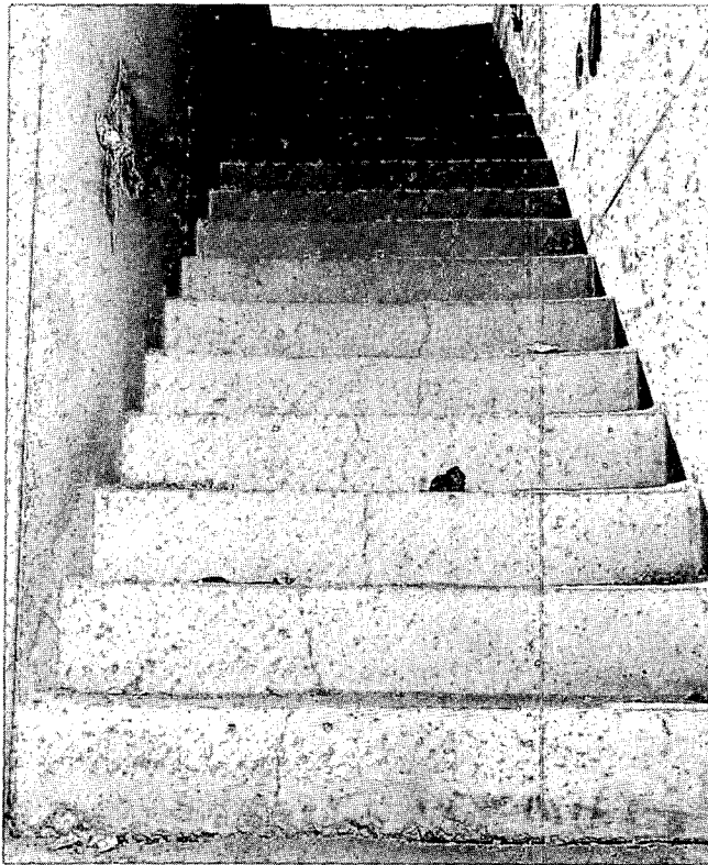
Fig. 3.71—Looking up stairs facing away from GZ (structure CAa). Note crack running up stairs and separation of construction joint.
