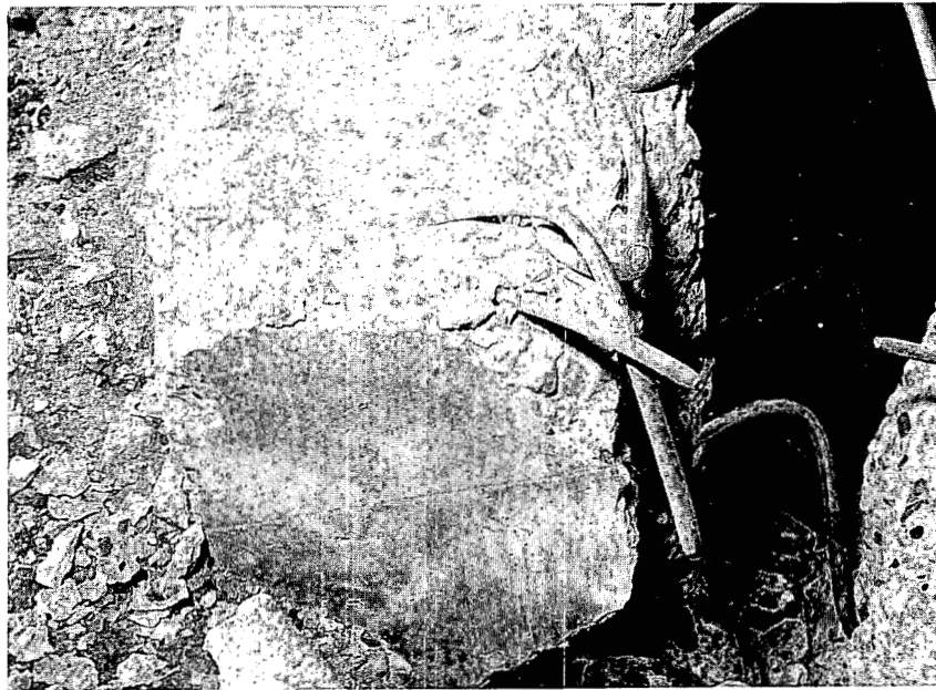
Fig. 3.22—Detail of exposed reinforcement after chipping at corner of interior wall and parapet facing toward GZ (structure RAa).
