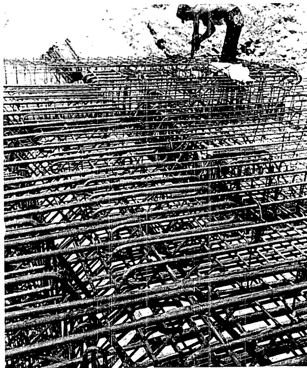
Fig. A.8—Detail of roof-slab reinforcement (structure RA) (May 8, 1957).
