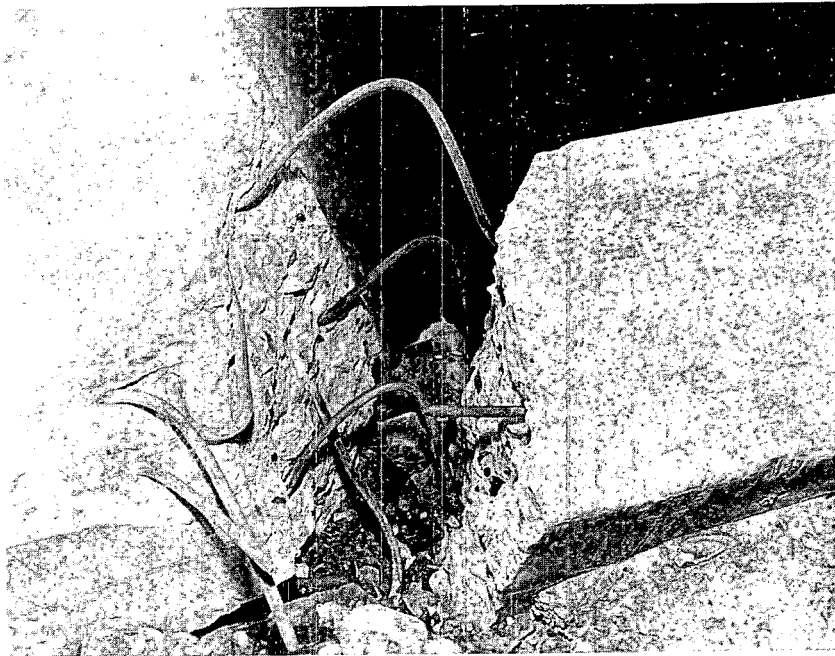
Fig. 3.19—Detail of crack at intersection of interior wall and parapet wall facing toward GZ (structure RAa).
