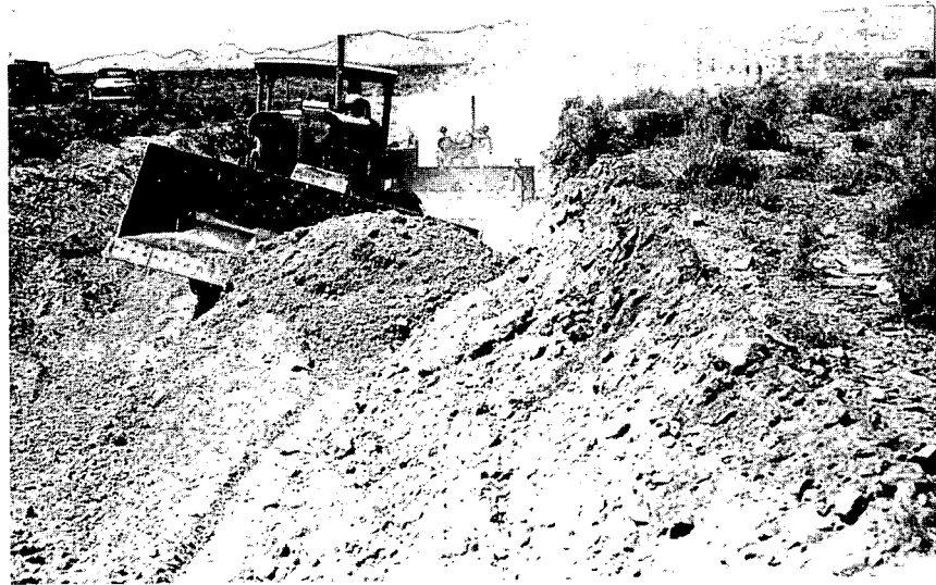
Fig. A.24—Use of blade rippers during excavation.
