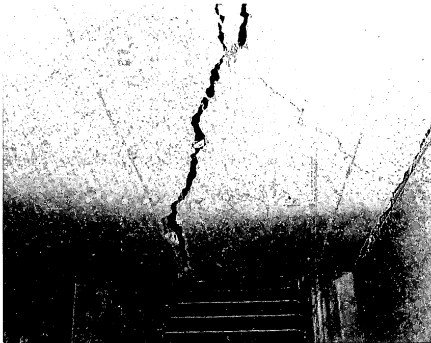
Fig. 3.9—Cracks along center of landing roof slab and at intersection with exterior wall (structure RAa).
