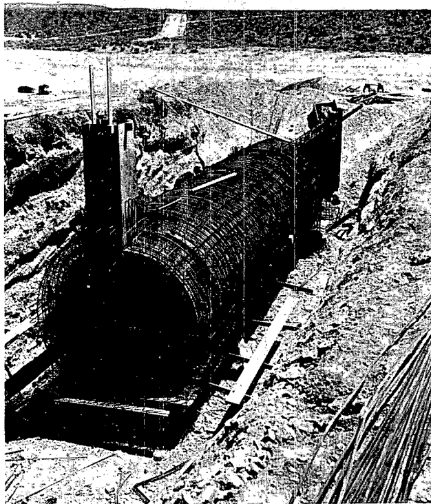
Fig. A.16—Reinforcement in place for main body of structure (structure CA) (June 18, 1957).
