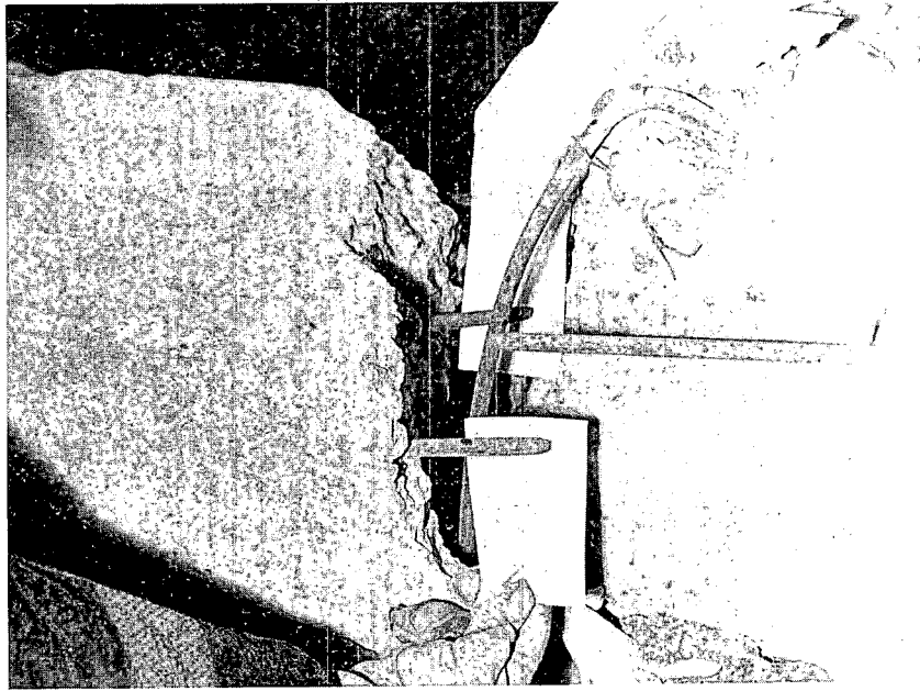
Fig. 3.18—Detail of necked-down reinforcement at intersection of exterior wall and parapet wall facing toward GZ (structure RAa).
