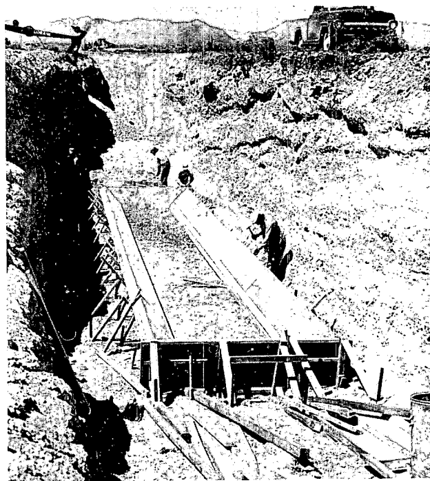
Fig. A.11—Erection of base-slab formwork (structure CA) (Apr. 25, 1957).
