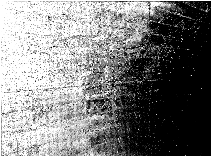
Fig. 3.77—Side of chamber facing away from GZ (structure CAb). Note survey point X-5, cracks, and horizontal cold joint.
