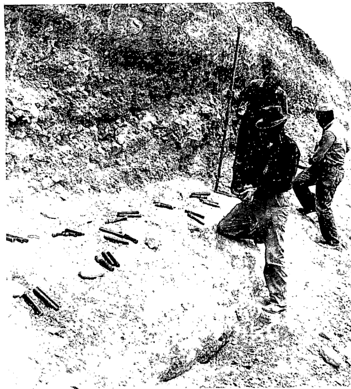
Fig. A.25—Preparation of dynamite for tamping into drill holes.
