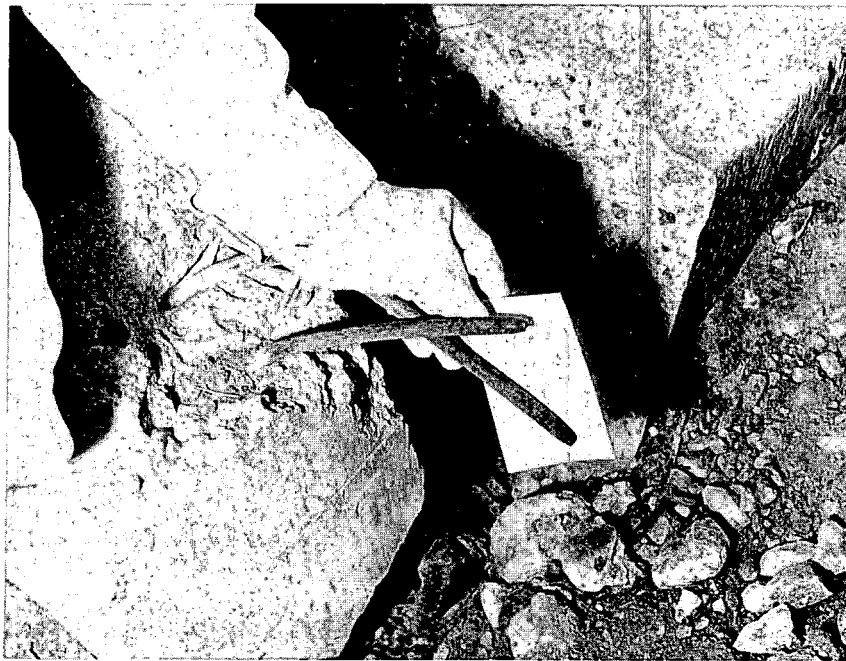
Fig. 3.20—Detail of necked-down reinforcement torn from parapet at interior wall (structure RAa).
