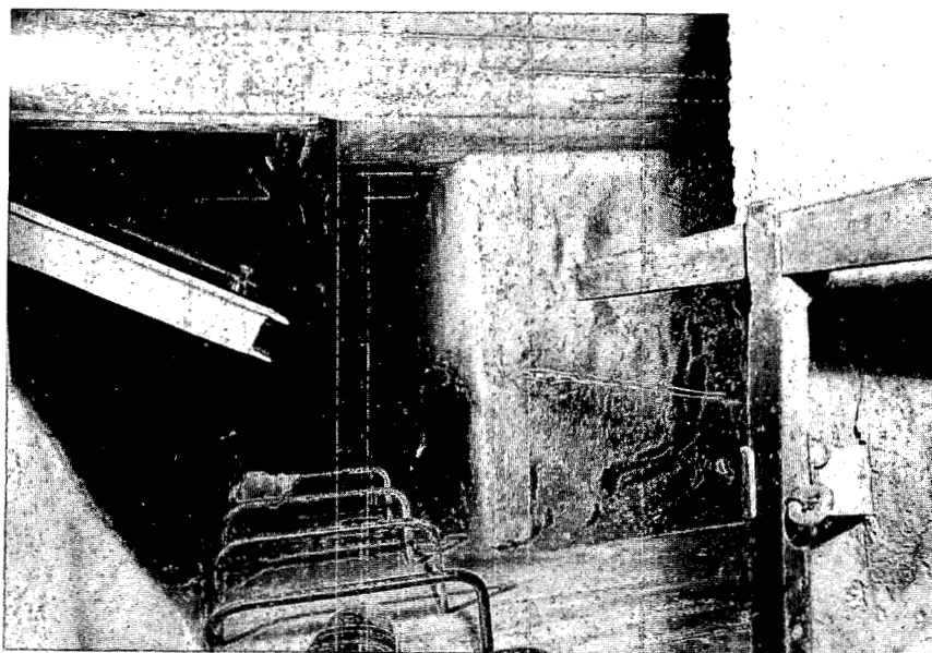
Fig. 1.18—Emergency exit blast door (structure CA).
