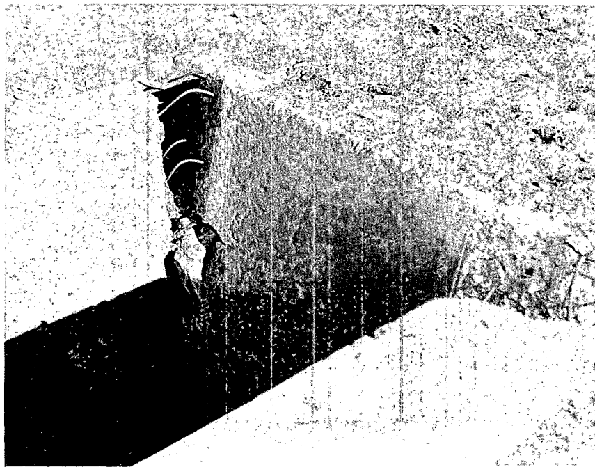
Fig. 3.15—Blast damage at intersection of interior wall and parapet wall facing toward GZ. (structure RAa).
