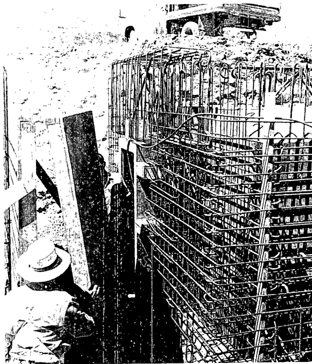
Fig. A.7—Erected formwork for entranceway walls and roof slab (structure RA) (May 4, 1957).
