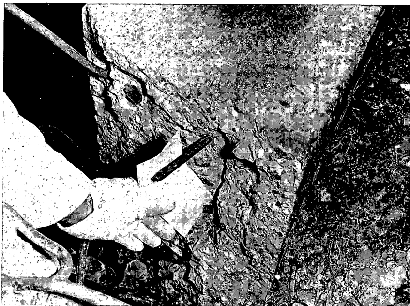
Fig. 3.21—Detail of necked-down reinforcement torn from interior wall at parapet (structure RAa).
