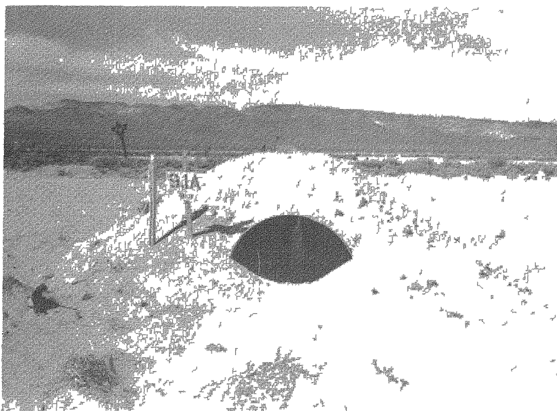
Fig. 2.12 Completed Structure B-3 with 2 Ft. of Earth Cover
