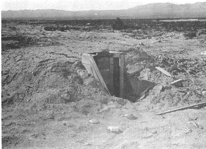
Fig. 4.1 Damage to Structure A-1 Due to Shot Baker (covered-trench below-grade)
