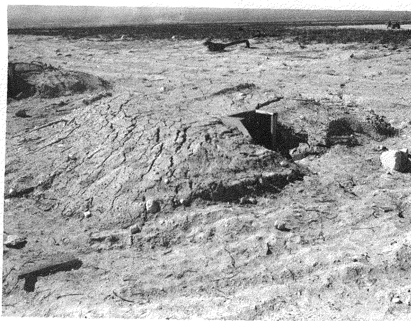
Fig. 4.7 Shelter A-14 After Shot Baker (below-grade lightened-frame)
