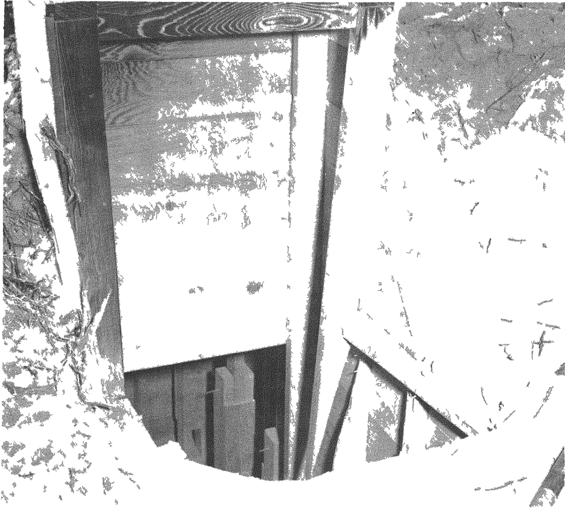
Fig. 4.5 Shelter A-5 After Shot Baker (below-grade lightened-frame)
