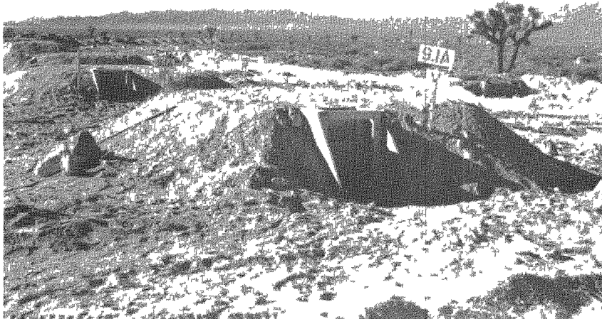
Fig. 2.5 Shelter A-1 Completed with 3 Ft. of Earth Cover (below grade)
