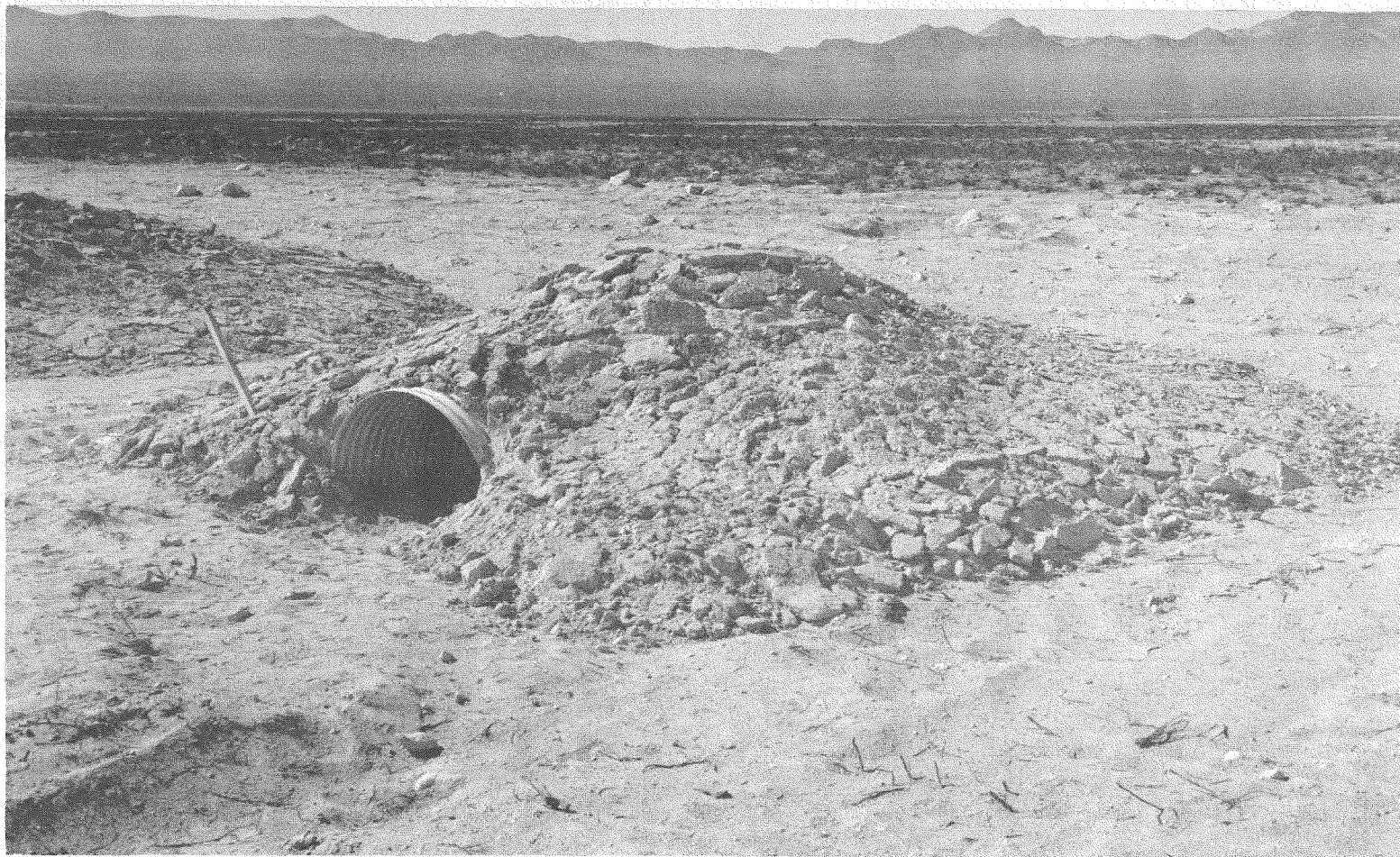
Fig. 4.14 Structure B-4 After Shot Baker (metal-arch, 16 gauge with 3 ft. of earth cover)
