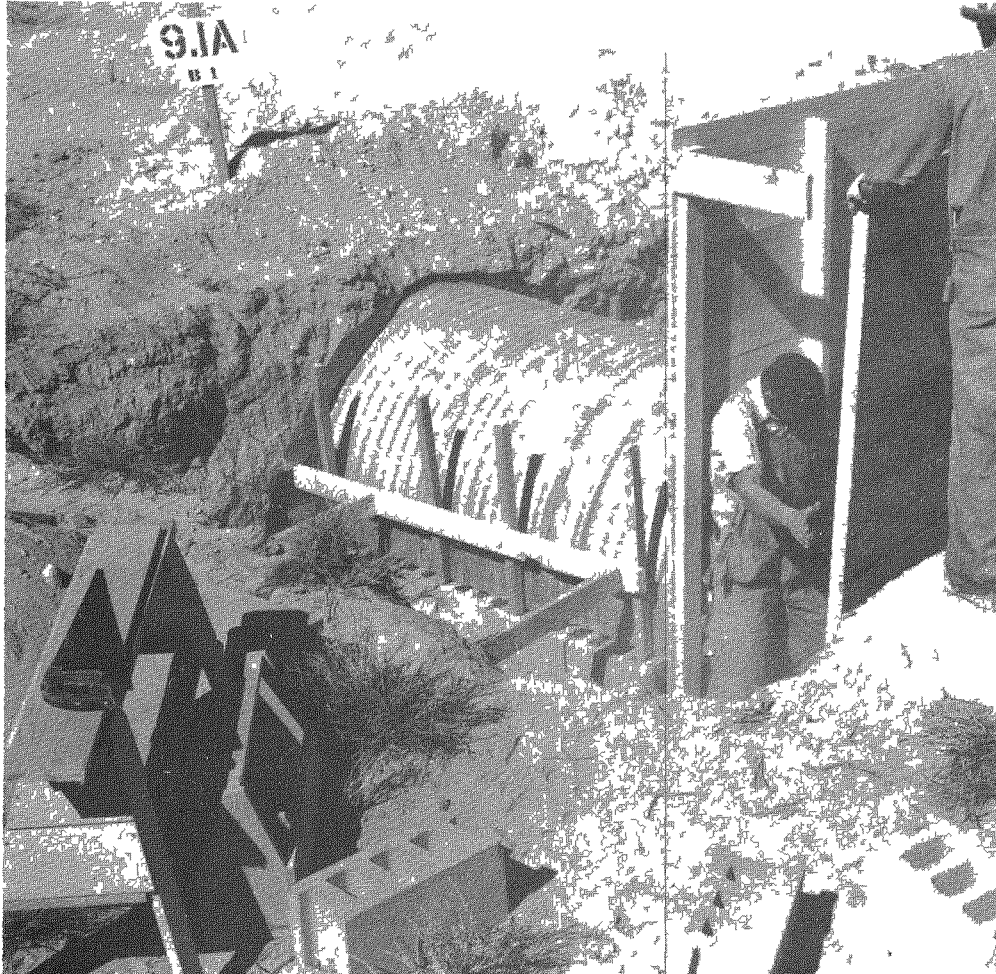
Fig. 2.8 Metal-arch Shelter B-1 Under Construction
