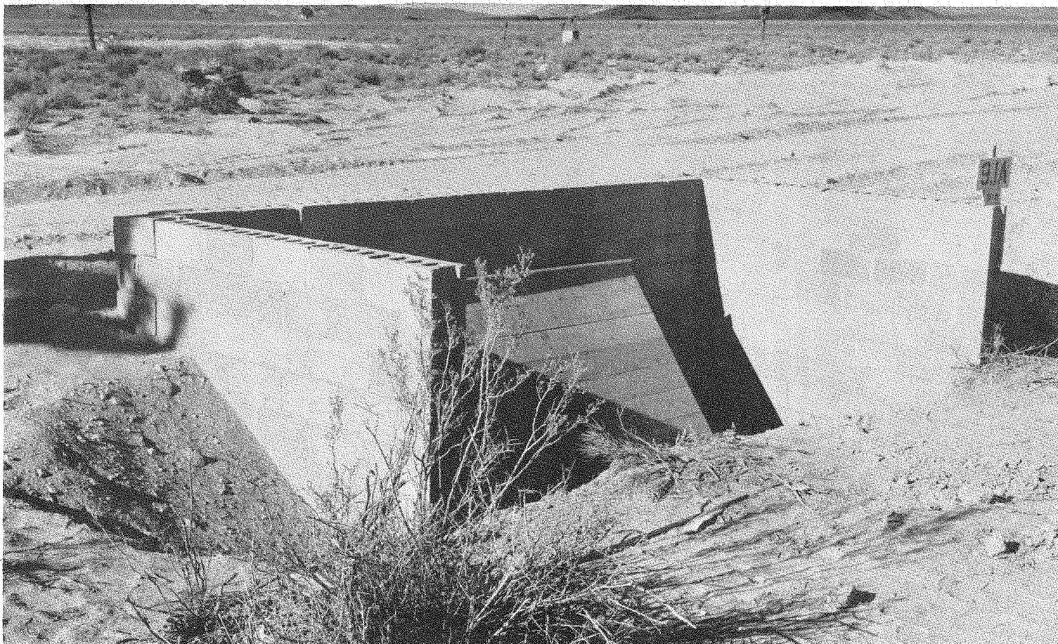
Fig. 2.17 Structure for Test of Basement Lean-to Shelter
