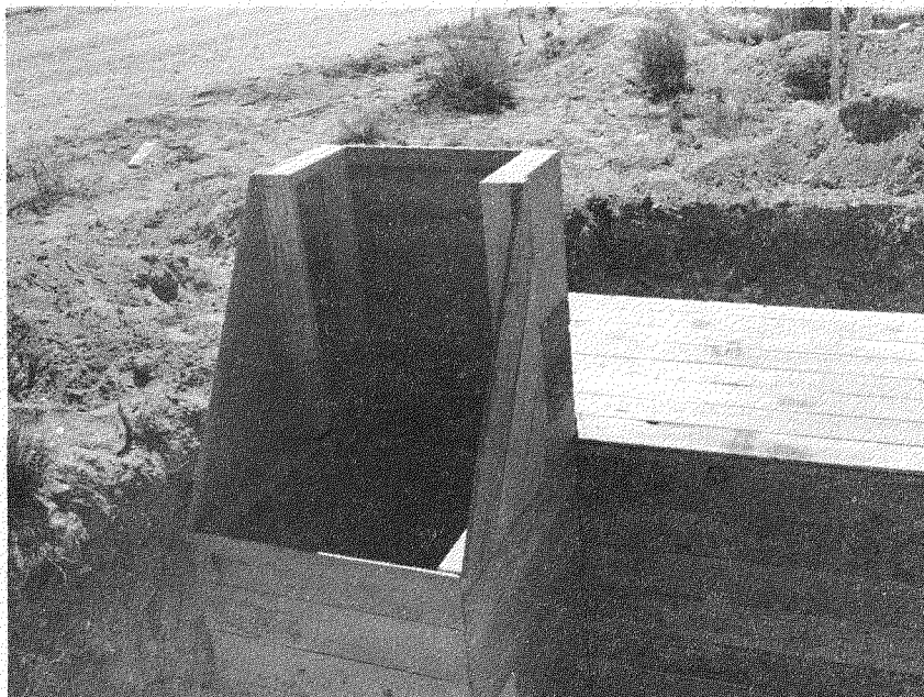
Fig. 2.3 Shelter Structure A-13 in Position Before Backfilling (below grade)
