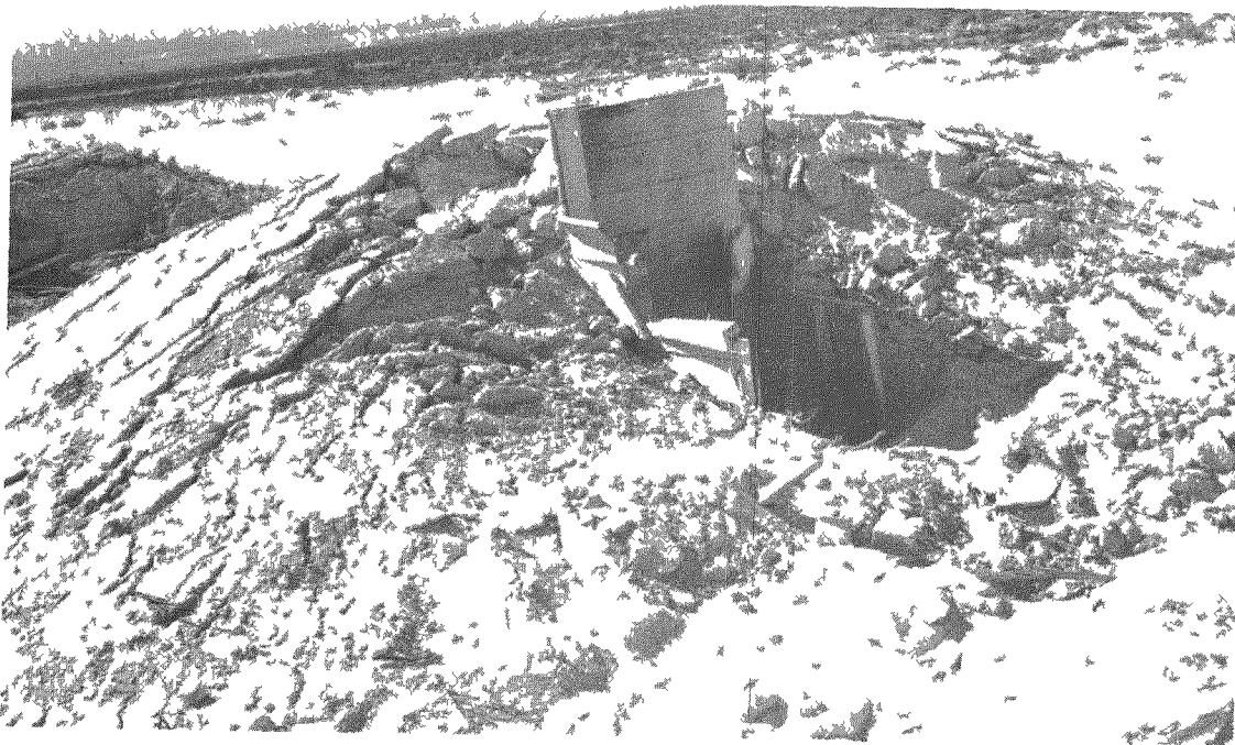
Fig. 4.12 Shelter A-17 After Shot Baker (partly above-grade lightened-frame)
