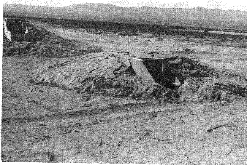
Fig. 4.6 Shelter A-8 After Shot Baker (below-grade lightened-frame)
