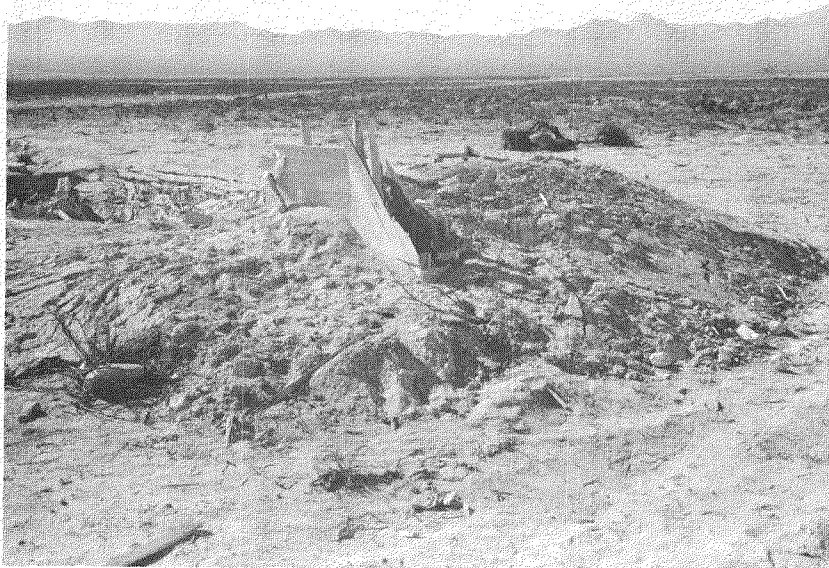
Fig. 4.17 Structure C-4 After Shot Baker (wood-arch)
