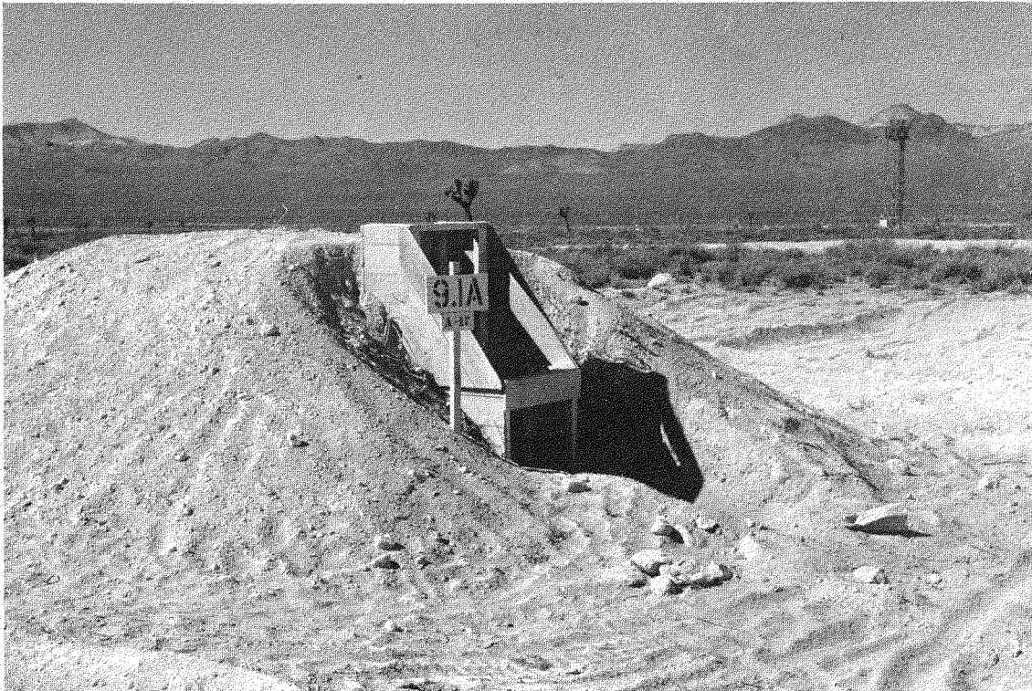
Fig. 2.7 Shelter A-17 Completed (partly above grade)
