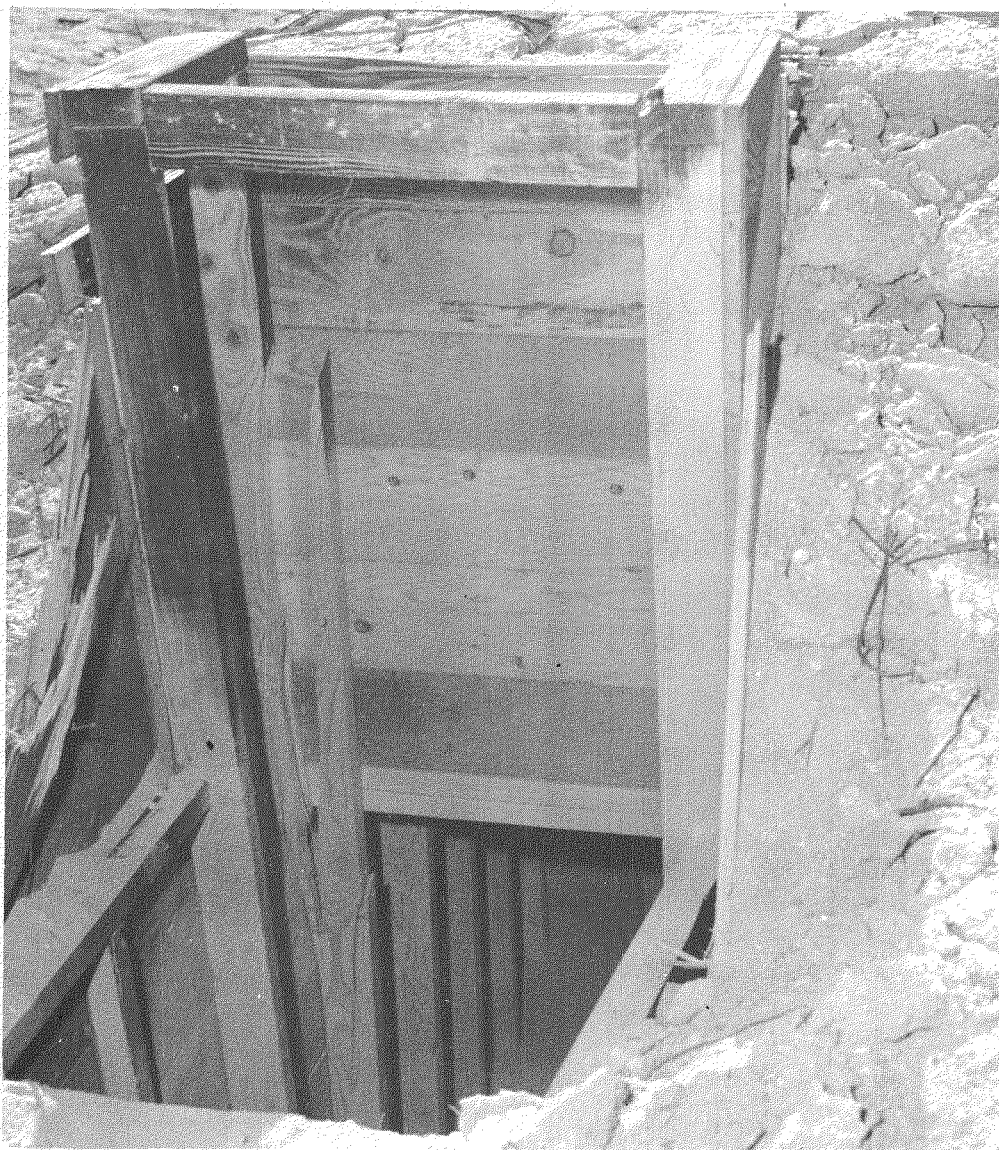
Fig. 4.8 Shelter A-15 After Shot Baker (below-grade lightened-frame)
