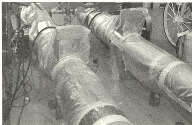
Fig. 4. 5-MW heat exchanger with sections isolated by polyethylene sheeting.
