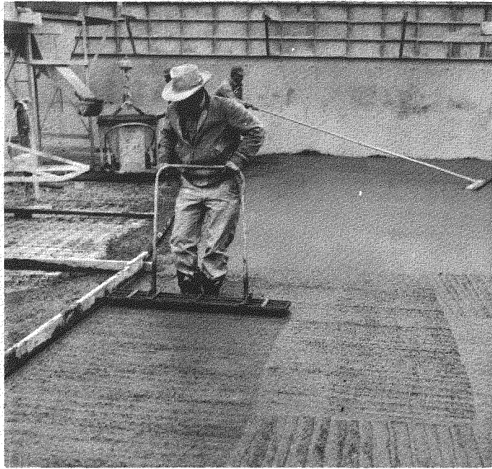
Fig. B.7—Puddling and finishing of floor slab.
