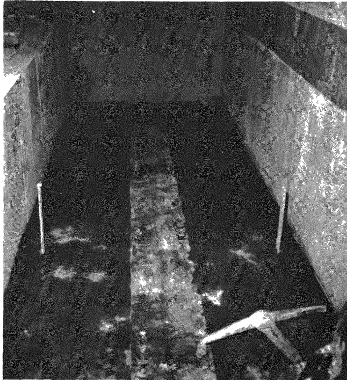
Fig. B.31—Rolling-door pit before installation of rail.
