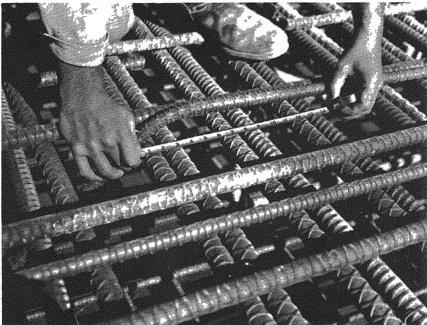
Fig. B.26—Reinforcement details at typical lap.
