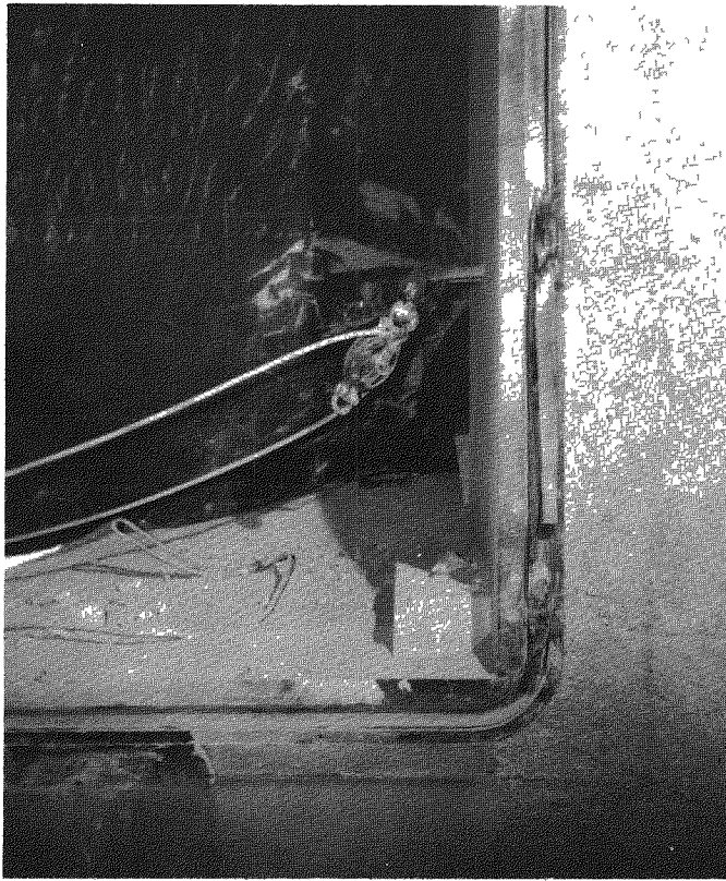
Fig. 3.11 — Damaged gasket at lower corner of door opening (postshot).
