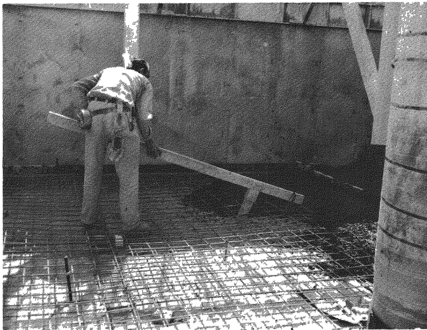
Fig. B.6—Placement of floor-slab concrete.
