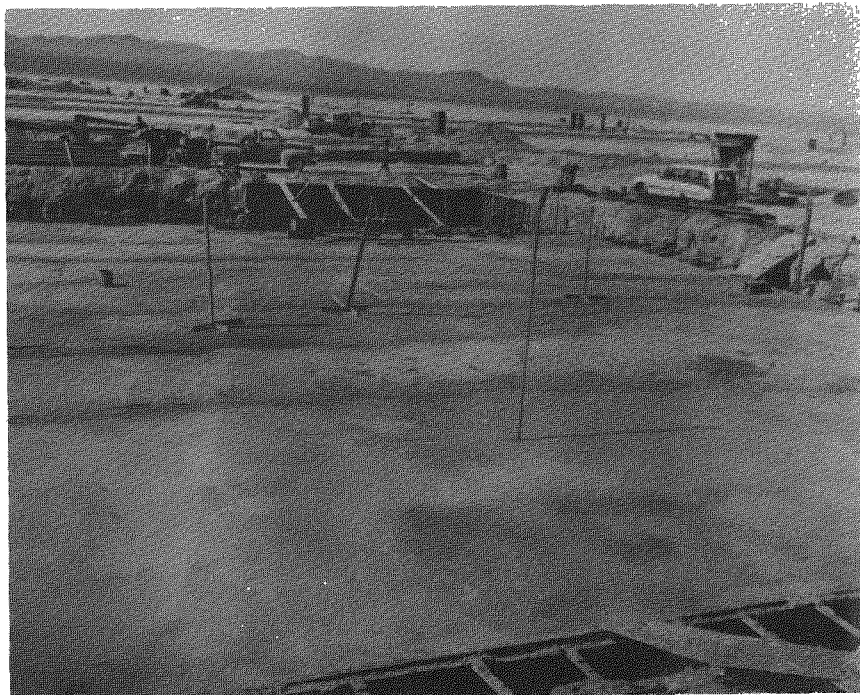
Fig. B.28—Roof-slab concrete placement completed. Note strip pattern of placement.
