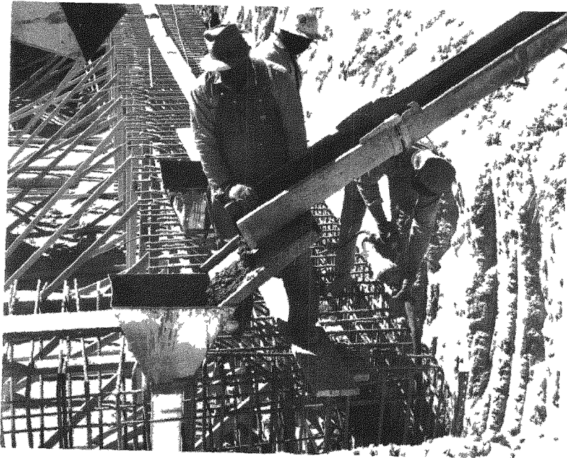
Fig. B.1—Placement of wall concrete using tremies.
