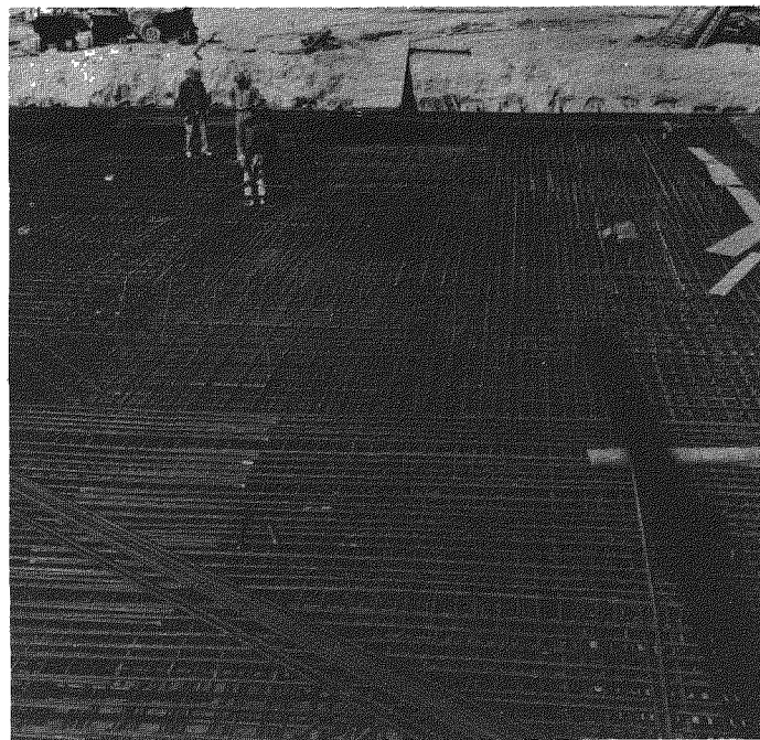
Fig. B.24—Partially completed roof-slab reinforcement.
