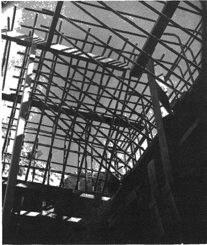
Fig. B.15—Partial roof-slab reinforcement at northeast corner.
