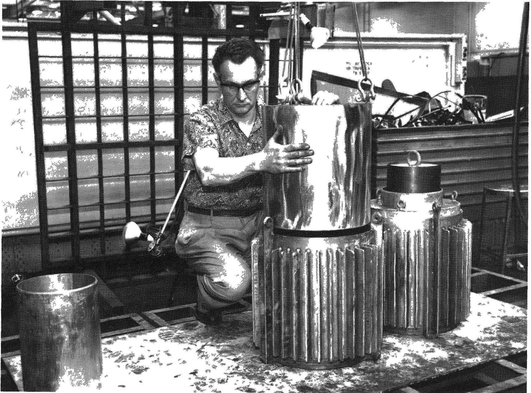
Fig. VI-3. Depleted-Uranium Shield Being Positioned for Insertion into Outer Hastelloy-C Shell
