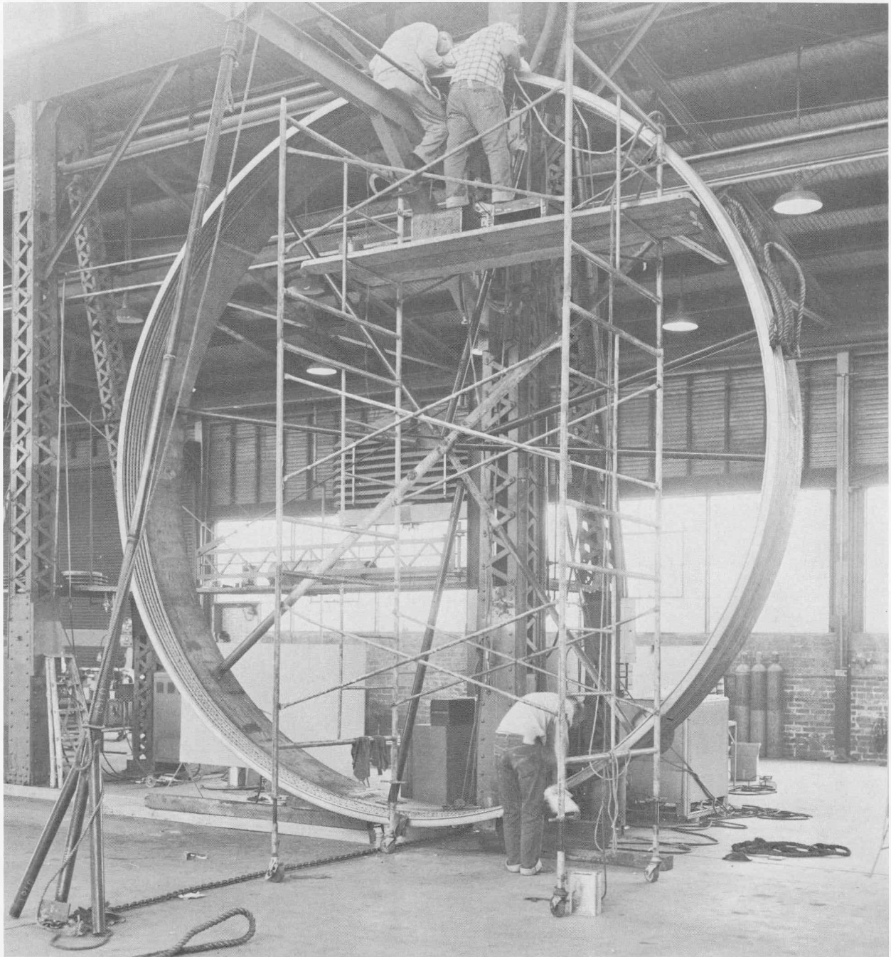
Figure 20. Reactor Vessel Bellows (welding of bellows convolutions in shop)
