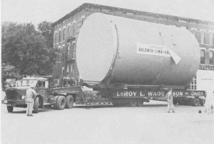
Figure 22. Reactor Vessel Transportation
