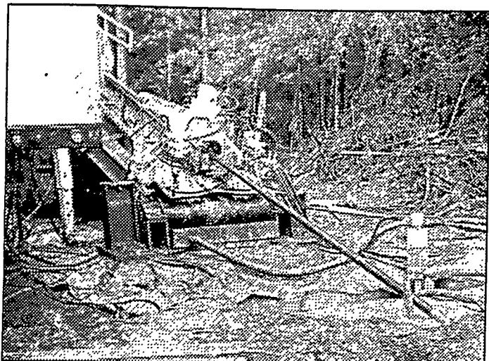
**HORIZONTAL WELLS:** an *in situ* bioremediation system that utilizes the installation of wells in the lateral planes of the subsurface to stimulate aerobic biodegradation of contaminants in underground water and soil.
