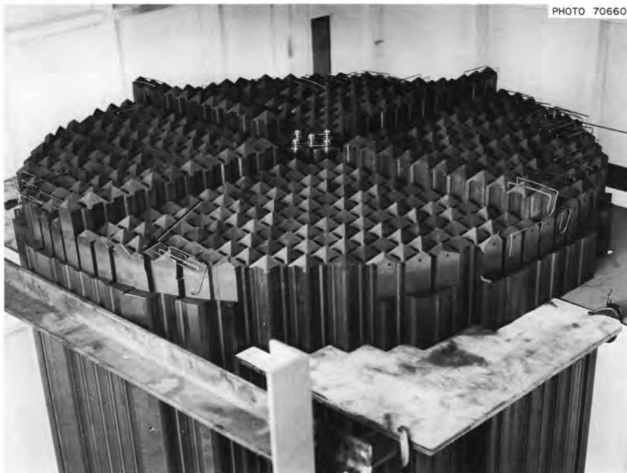
Fig. 1.6. Core graphite during assembly, before installation of retaining rings and centering bridge. Arrow points to piece similar to one found broken on top of core.
