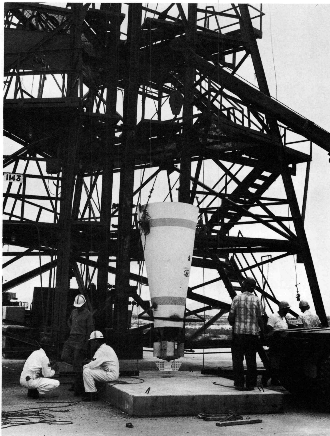
Figure 12. Drop-Tower Test, Pump-End Impact
