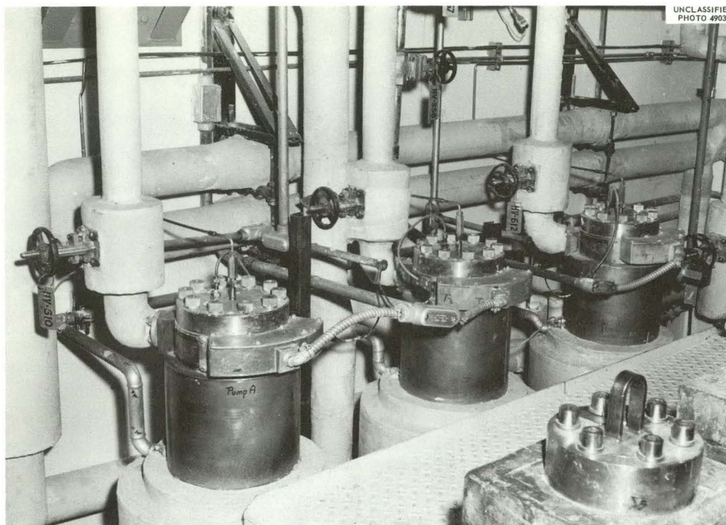
Fig. 23. Main Circulating Pumps with Installation Complete.
