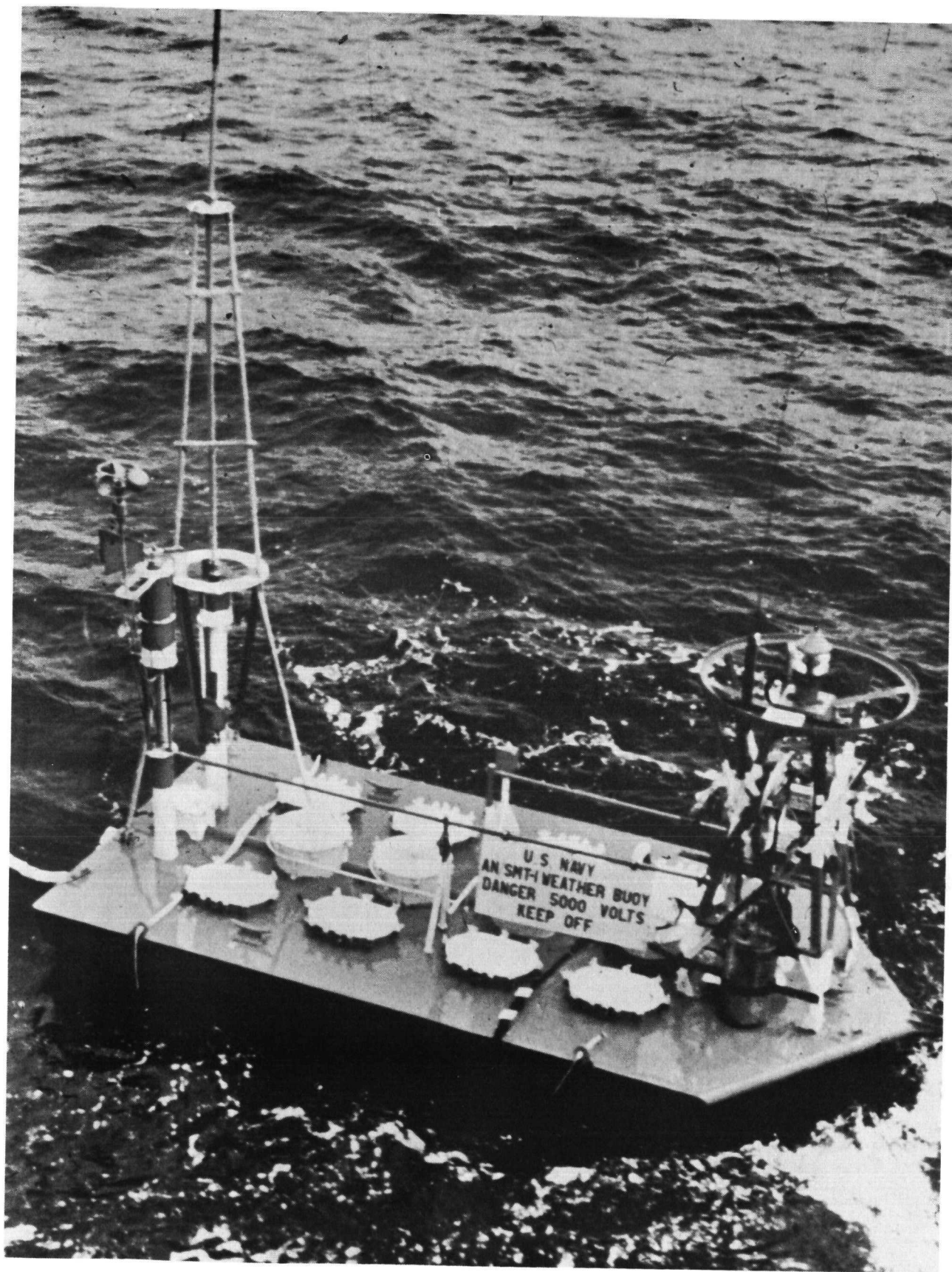
SNAP 7D U. S. Navy Floating Weather Station with Sr-90 Fueled Generator
