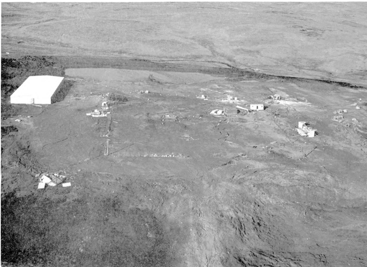
FIG. 6-3 (Above) D+T DAY VIEW OF THE SGZ AREA, LOOKING TO THE NORTHWEST
