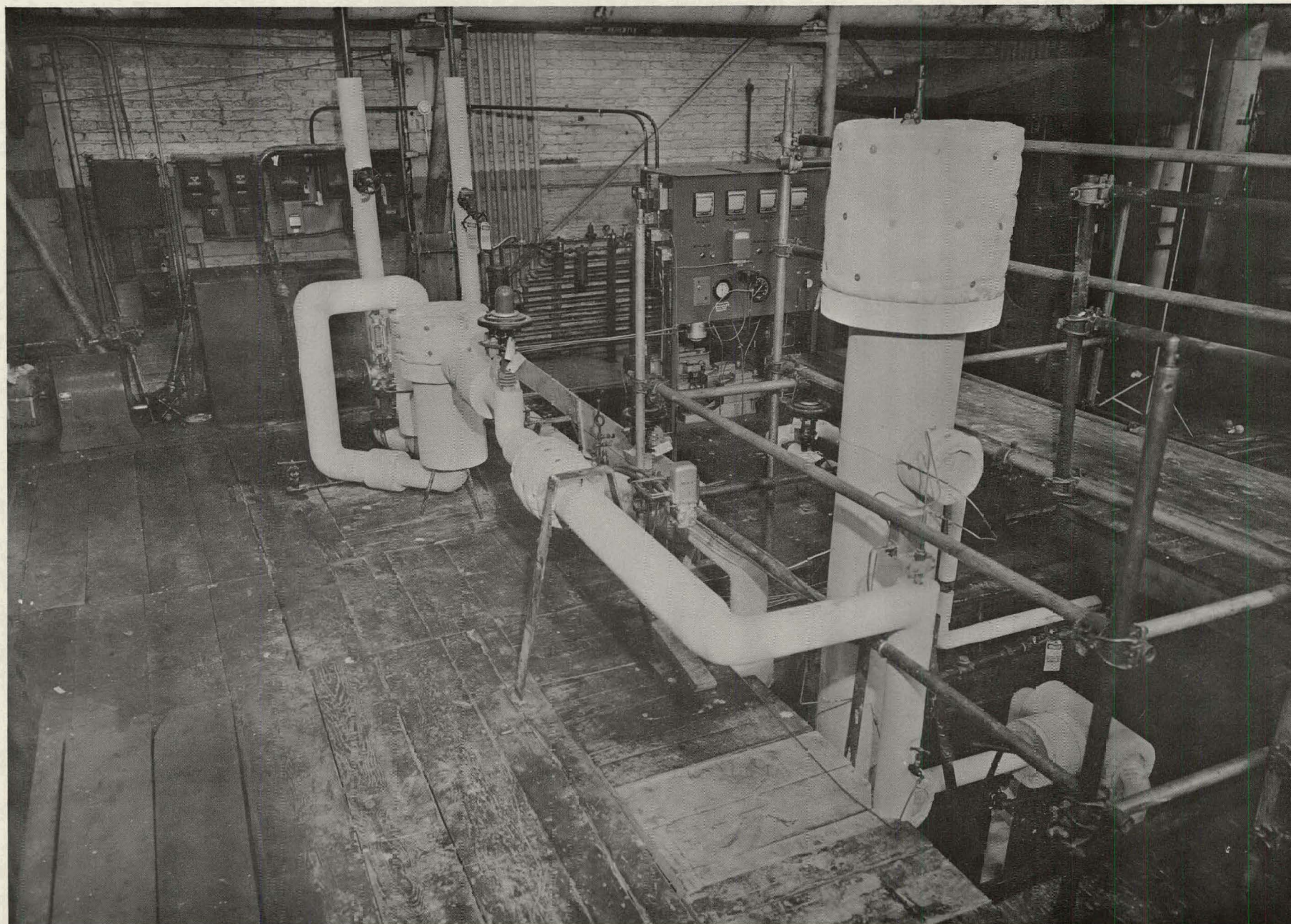
Fig. 1.2...Corrosion-Erosion Loop (212195)
