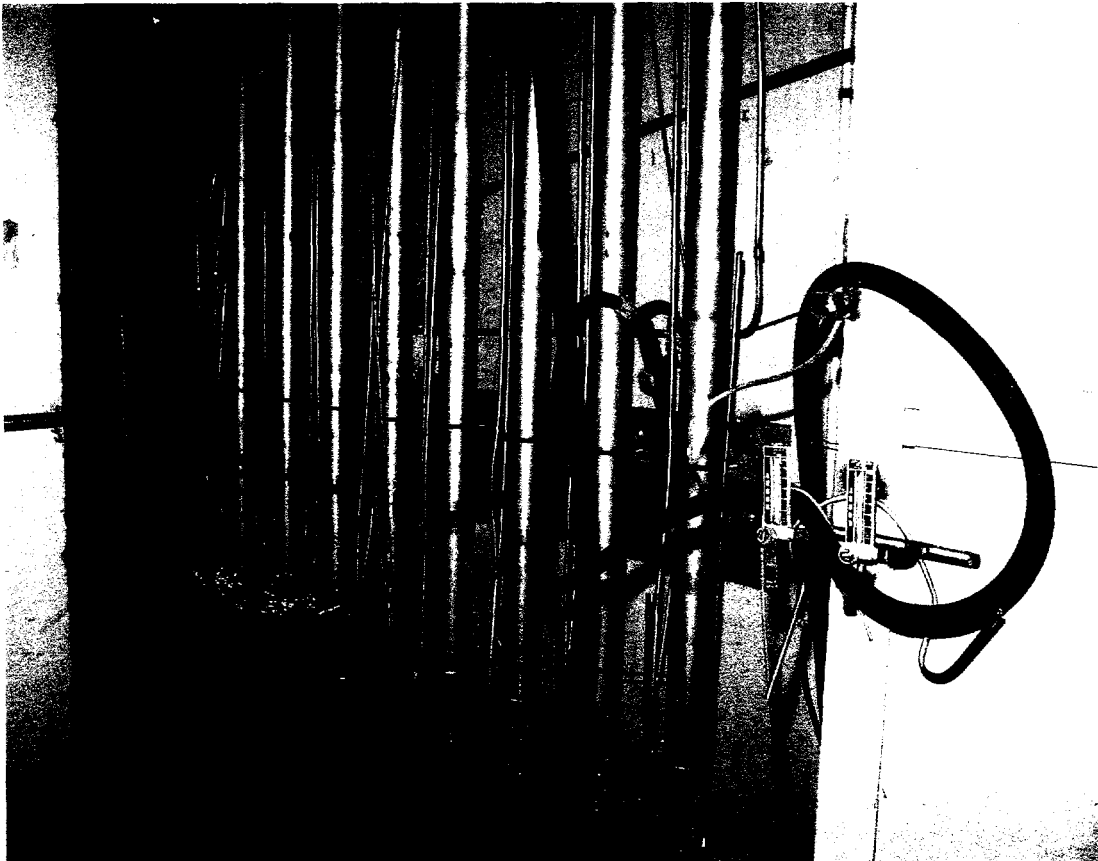
Fig. 37. Vertical configuration of tanks for the storage of concentrated solutions of fissile material. These vessels were used in the first reprocessing pilot plant in the United States.
