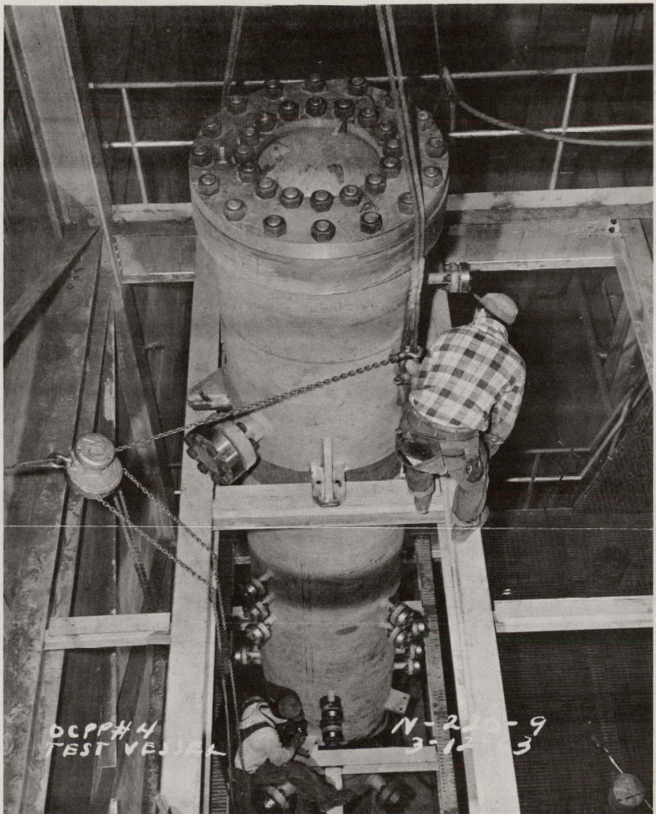
Figure 45 - Pressure Vessel Installation
