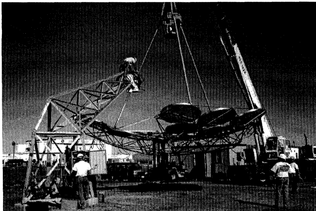
Figure 3. Photograph taken while the mirrors support structure, with mirrors attached, was being lifted to mate with the declination beam and drive assembly.
