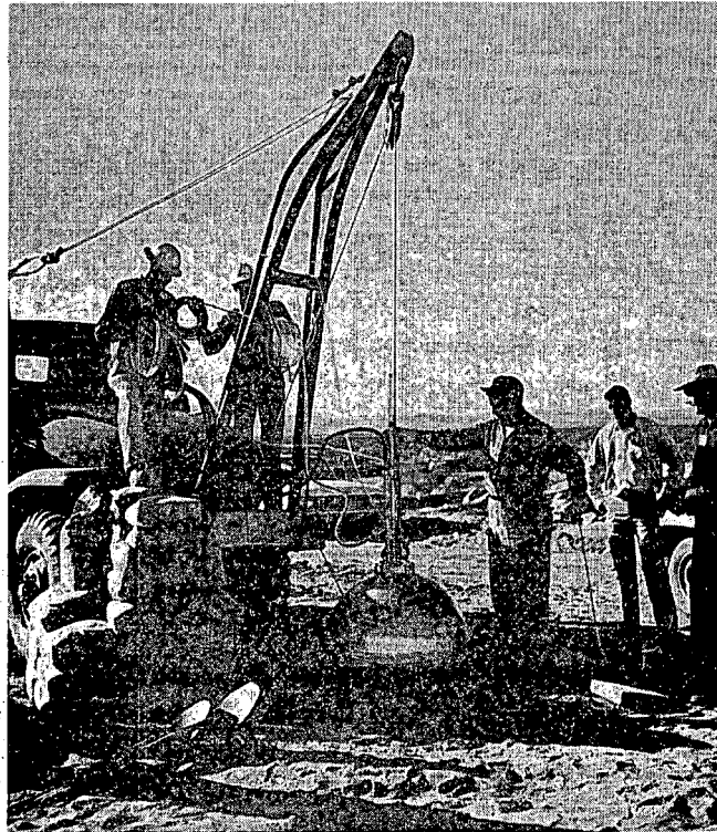
Figure 2.3 H. E. sphere and emplacement hole.
