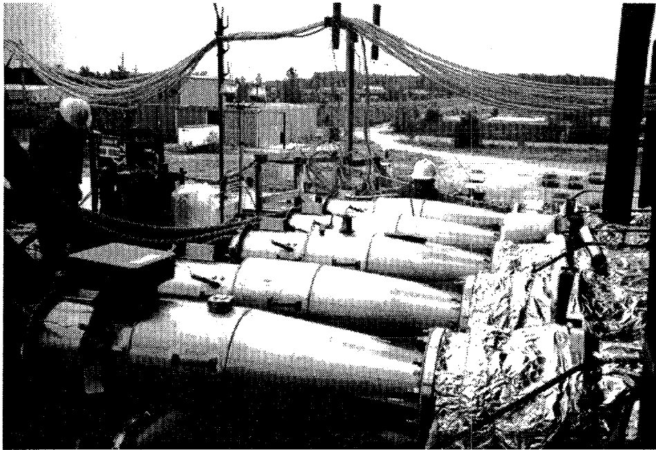
Figure 6. Cooperheat 6,000,000 BTU/hour Environmental Propane Burners.
