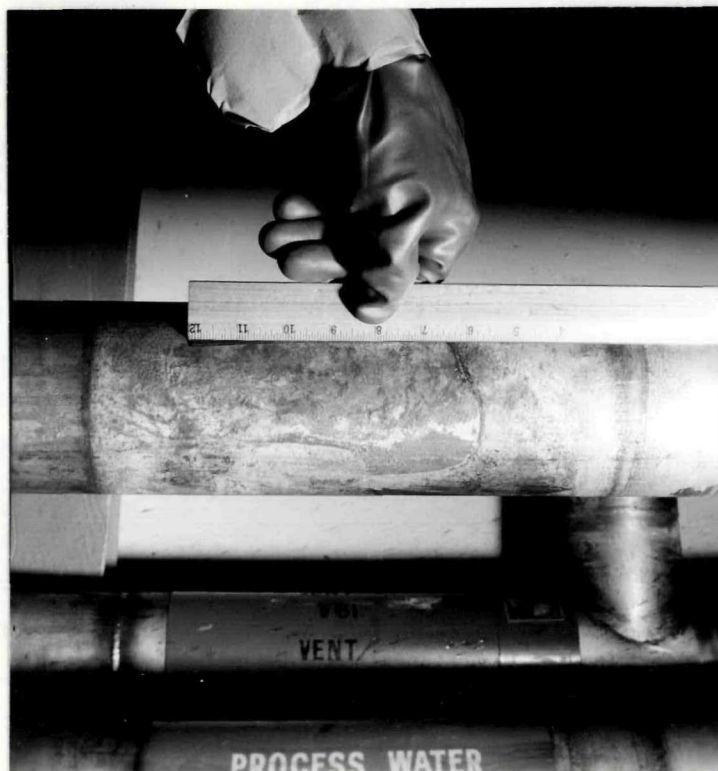
FIGURE 1. STRESS CORROSION UNDER LABELS. Atmospheric moisture concentrates chlorides under labels. Rusty corrosion products indicate beginning of attack. Careful inspection is required to detect cracks.
