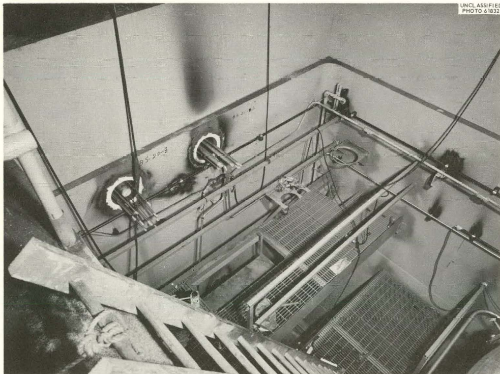
Fig. 10.2. South End of Cell B, Showing Piping Penetrations.
