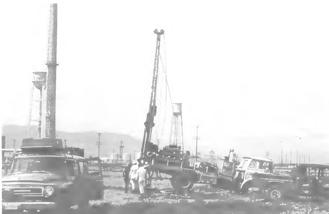
Fig. II-6 Auger equipment drilling a sample hole beneath the pond.
