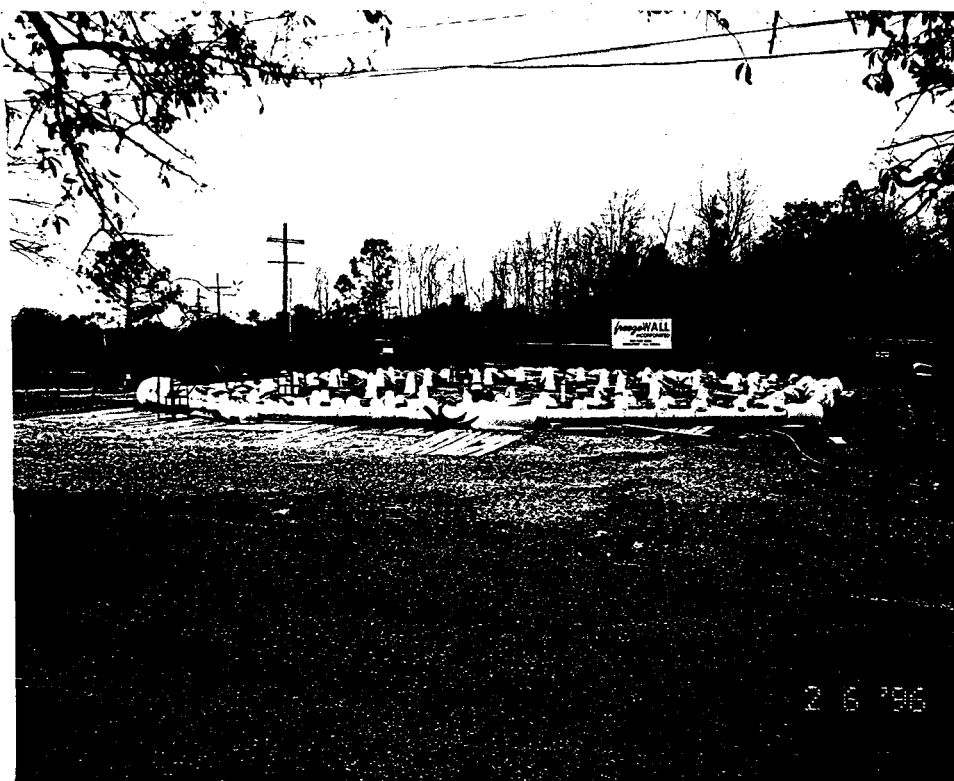
Fig. 3 A cylindrical freeze curtain was constructed around the sinkhole, extending 6 m into salt, so that groundwater inflow was inhibited, if not stopped. A hydrologic monitoring system consisting of piezometers below the top of salt and brine injection within the the sinkhole throat confirmed the integrity of the mitigation.
