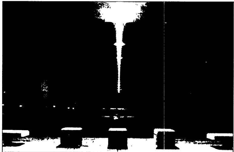
The sulfur lamp installation outside of DOE's Forrestal Building produces 4 times as much light at 1/3 the cost of conventional lighting.
