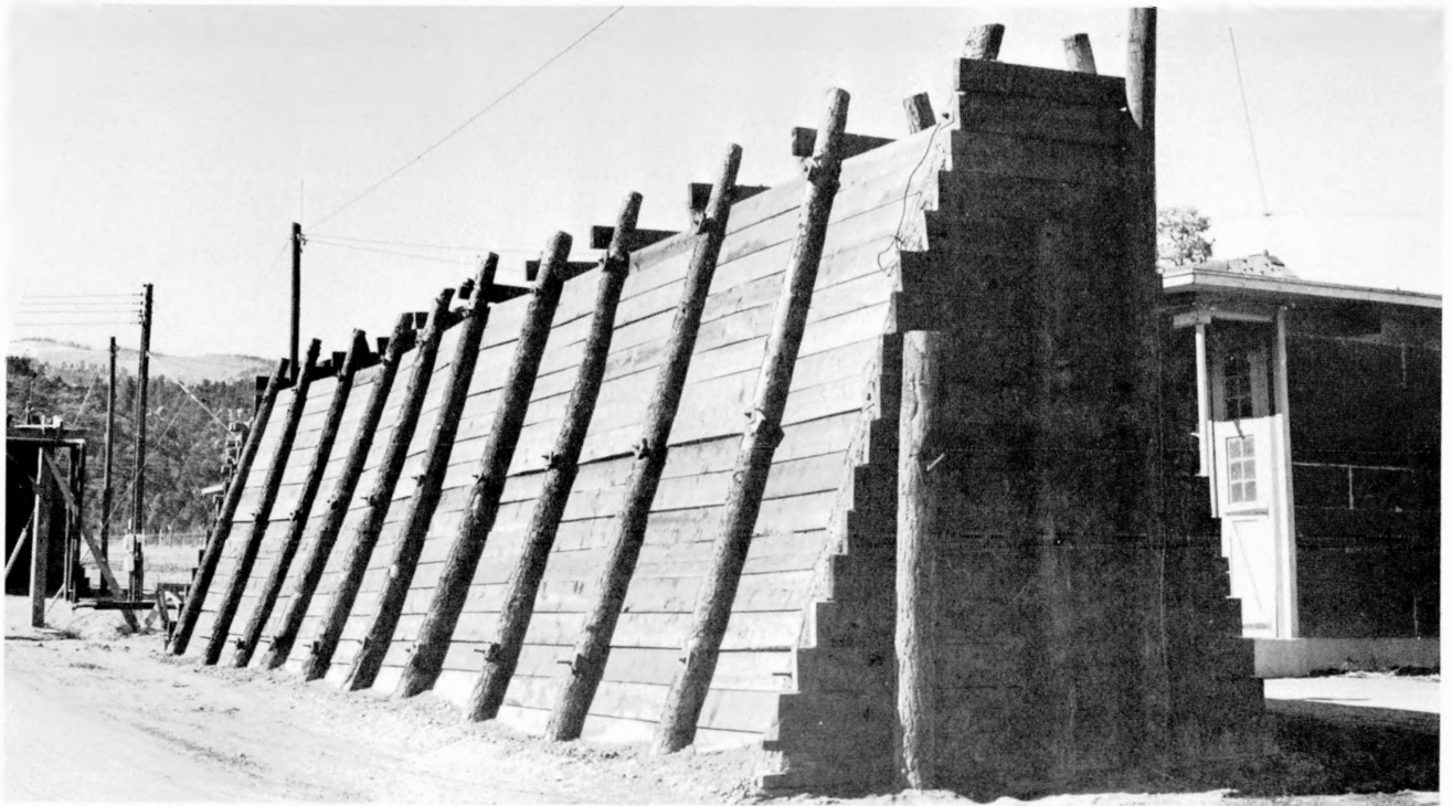
Fig. 29. Wooden and earth-filled barricade near Building S-24, S Site.
