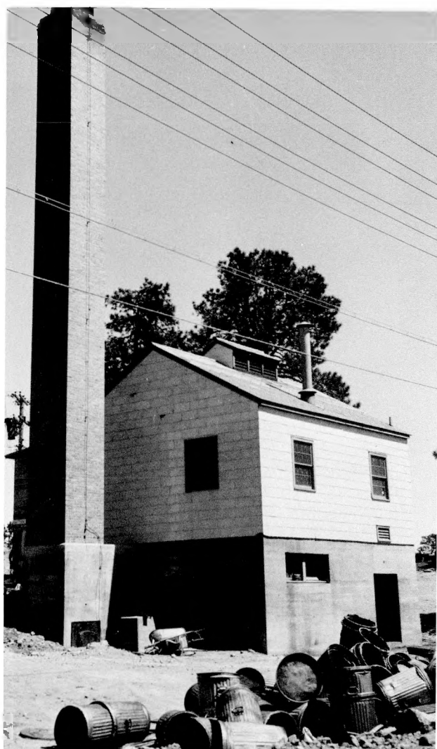
Fig. 84. Incinerator, 5-ton capacity.
