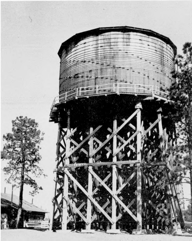
Fig. 7. The 250,000-gal tank. The building in the left center is an original shop of the Los Alamos Ranch School which was converted into the Housing and Express Office.
