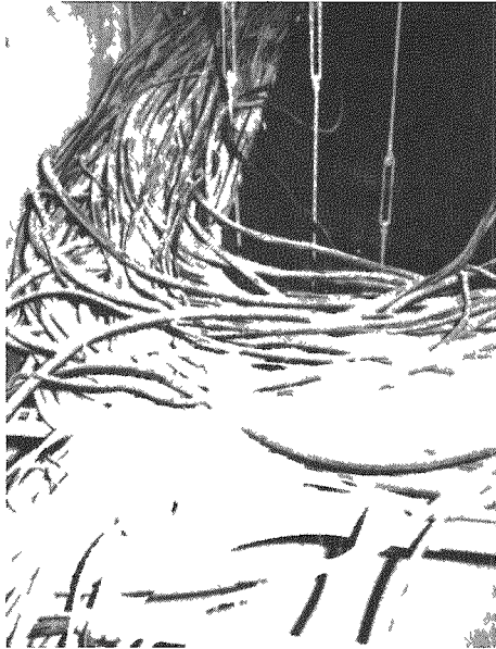
FIG. 24 CROWDED CABLE TRAY IN PRIMARY INERT GAS BUILDING BEFORE CABLE REPLACEMENT AND REROUTING
