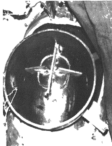
FIG.3 LOCATING PLATES WELDED TO PATCH
