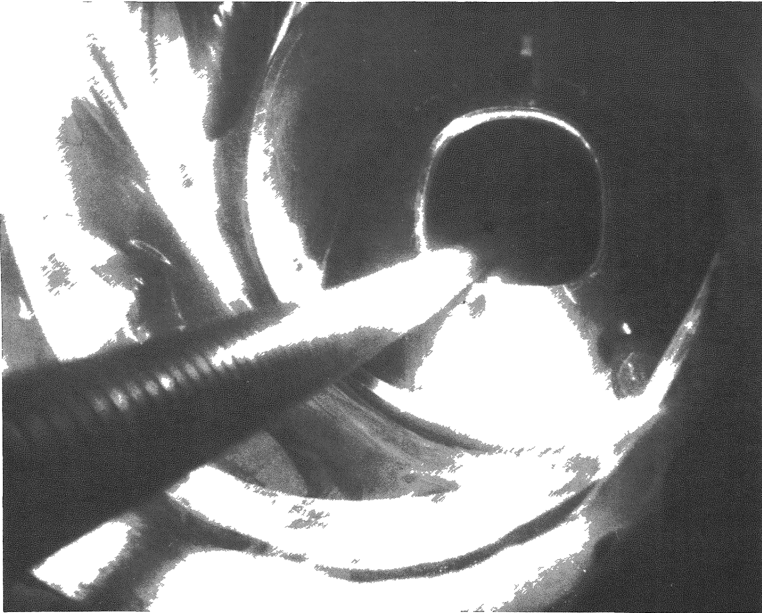
FIG.7 OBJECT-RETRIEVAL DEVICE CABLE INSERTED THROUGH PRIMARY ELBOW PENETRATION
