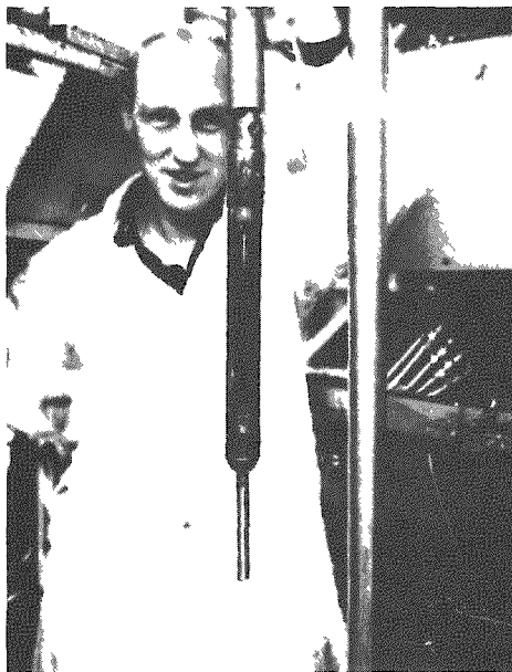
FIG.8 FIVE-INCH LENGTH OF ROD WELDED TO OLD ARTICULATED LAMP TO MANEUVER OBJECT
