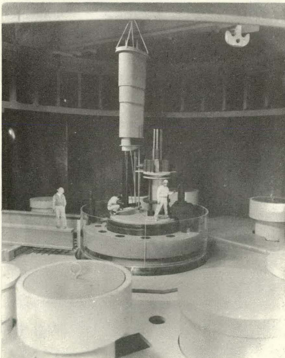
INSTALLATION OF OFFSET HANDLING MECHANISM
