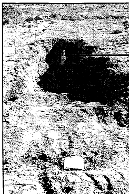
Figure 56. Excavation for Foam Block at Main Pad Area (C. T. Coffin is about 5' 8" tall for comparison)
