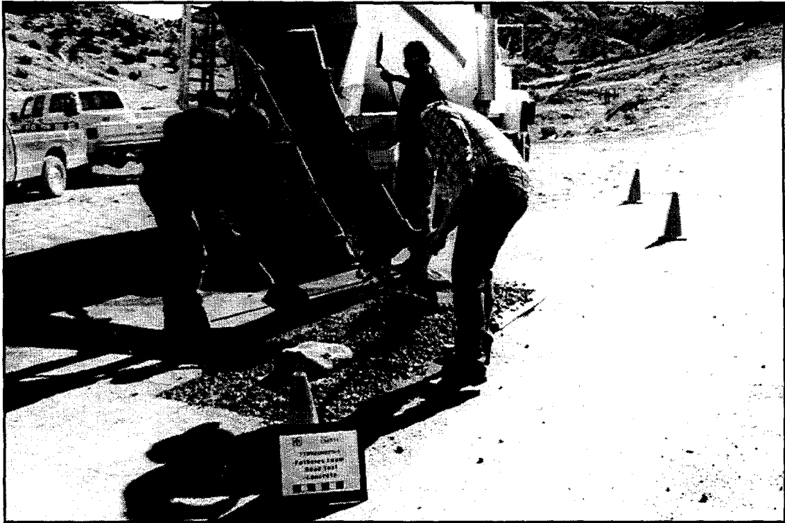
Figure 85. Concrete Road Experiment Samples Being Backfilled (note the large rocks holding blocks from floating up out of position)
