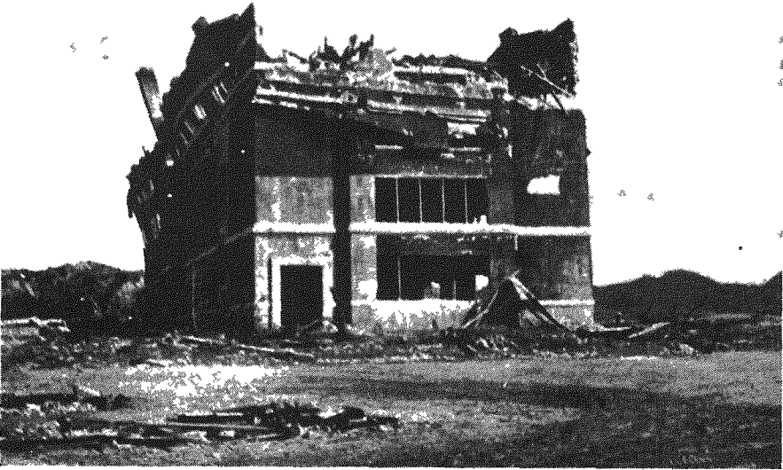
Photo No 5 NAGASAKI Reinforced concrete school with a timber roof, 500 yds from the centre of damage, which is to the right of the photograph. The upper part of the long wall further from the explosion has been bent over, partly by a thrust through the roof from the other long wall and partly by wind suction This is a typical case of "mass distortion." See paragraphs 15 and 22.
