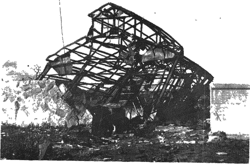
Photo No. 11. HIROSHIMA. Small steel framed shed \frac{1}{4} mile from the centre of damage, showing the distortion of the entire framework, with the building leaning away from the explosion. See paragraphs 22 and 32.
