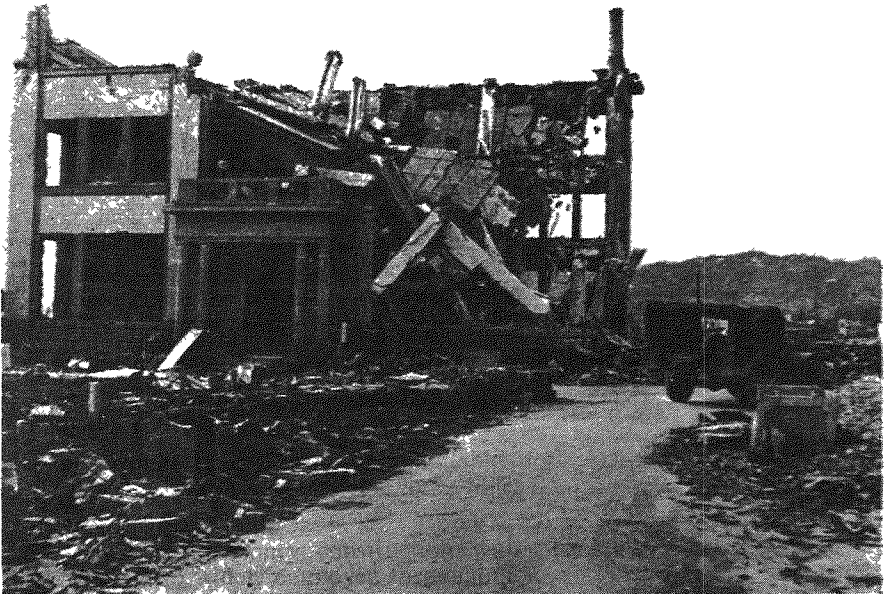
Photo No. 8. HIROSHIMA. Reinforced concrete building 200 yds. from the centre of damage, which is to the right. The blast from the bomb forced the roof slab down, the slab shearing round the column heads, leaving the internal columns projecting through the debris. Few concrete buildings failed in this way. See paragraph 24.
