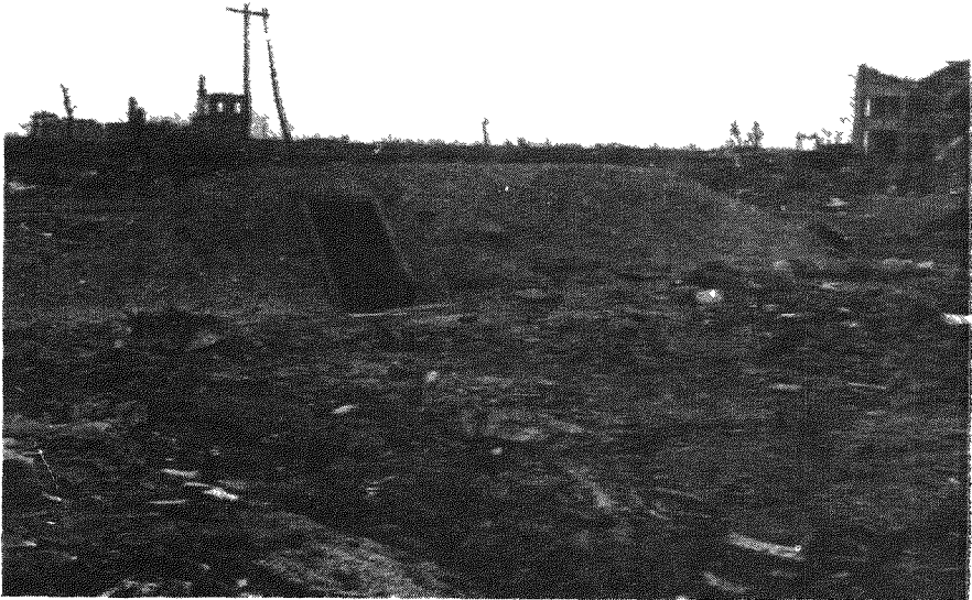
Photo No. 17. HIROSHIMA. Typical, part below ground, earth-covered, timber framed shelter 300 yds. from the centre of damage, which is to the right. In common with similar but fully sunk shelters, none appeared to have been structurally damaged by the blast. Exposed woodwork was liable to "flashburn." Internal blast probably threw the occupants about, and gamma rays may have caused casualties. See paragraph 40.
