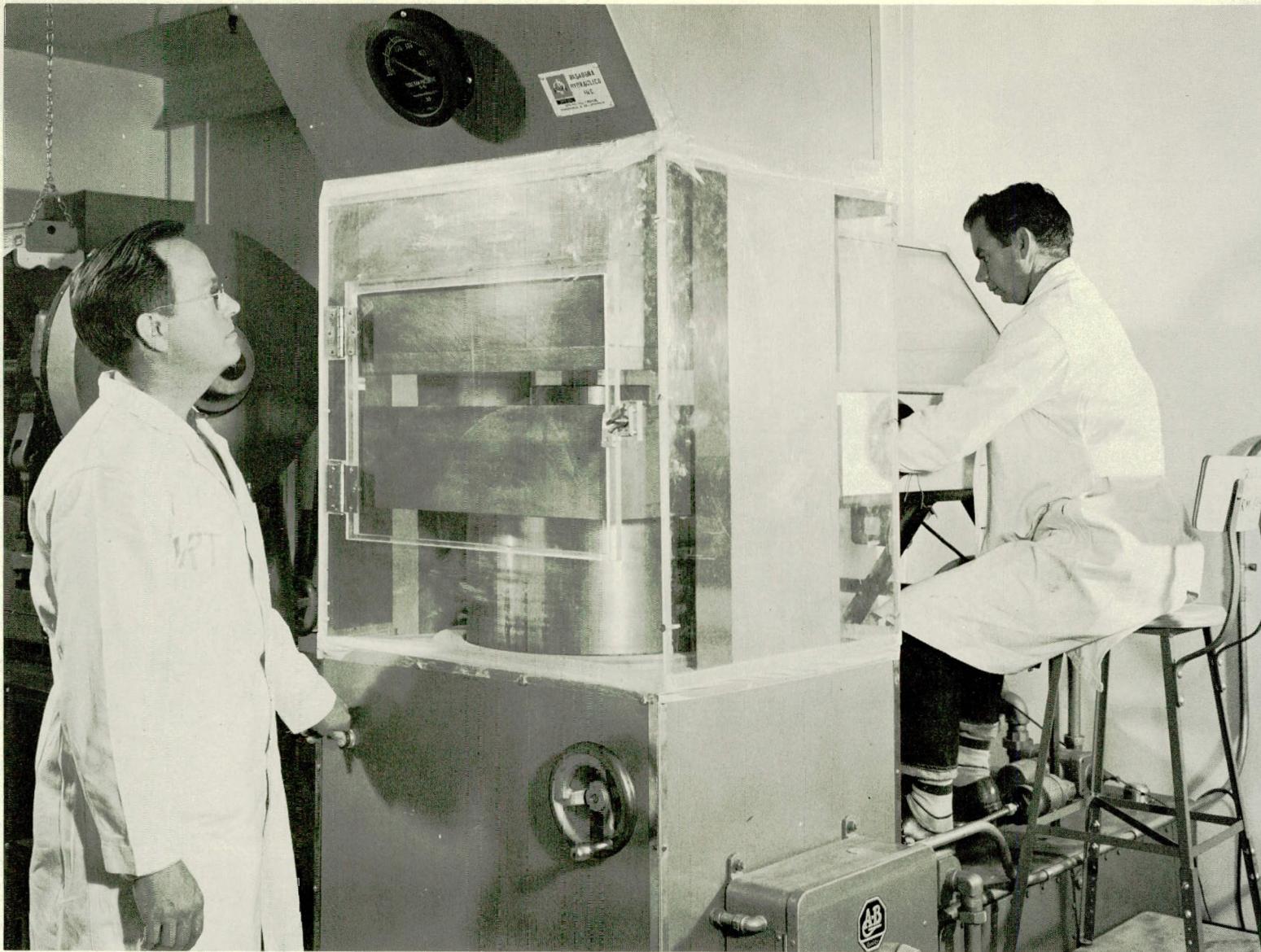
Fig. 8. Pressing Compacts for Fuel Core
